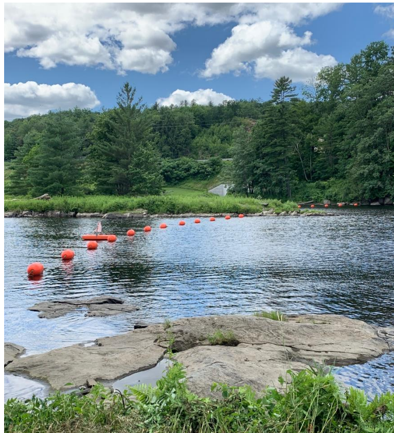
View of Boat Safety Cable Upstream of Dam
