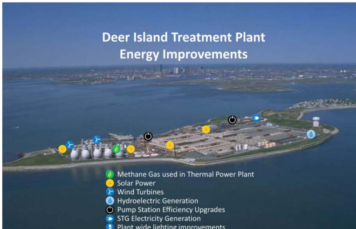
Figure 1: View of Deer Island Treatment Plant and Location of Deer Island Hydroelectric Project
