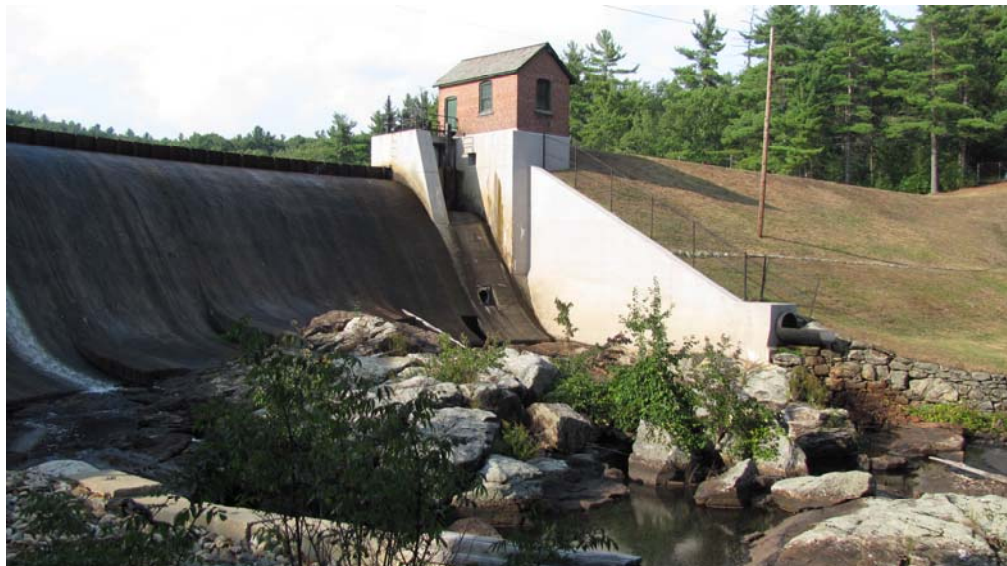
Figure 2 – Crocker Dam Downstream Face (Right Side)
