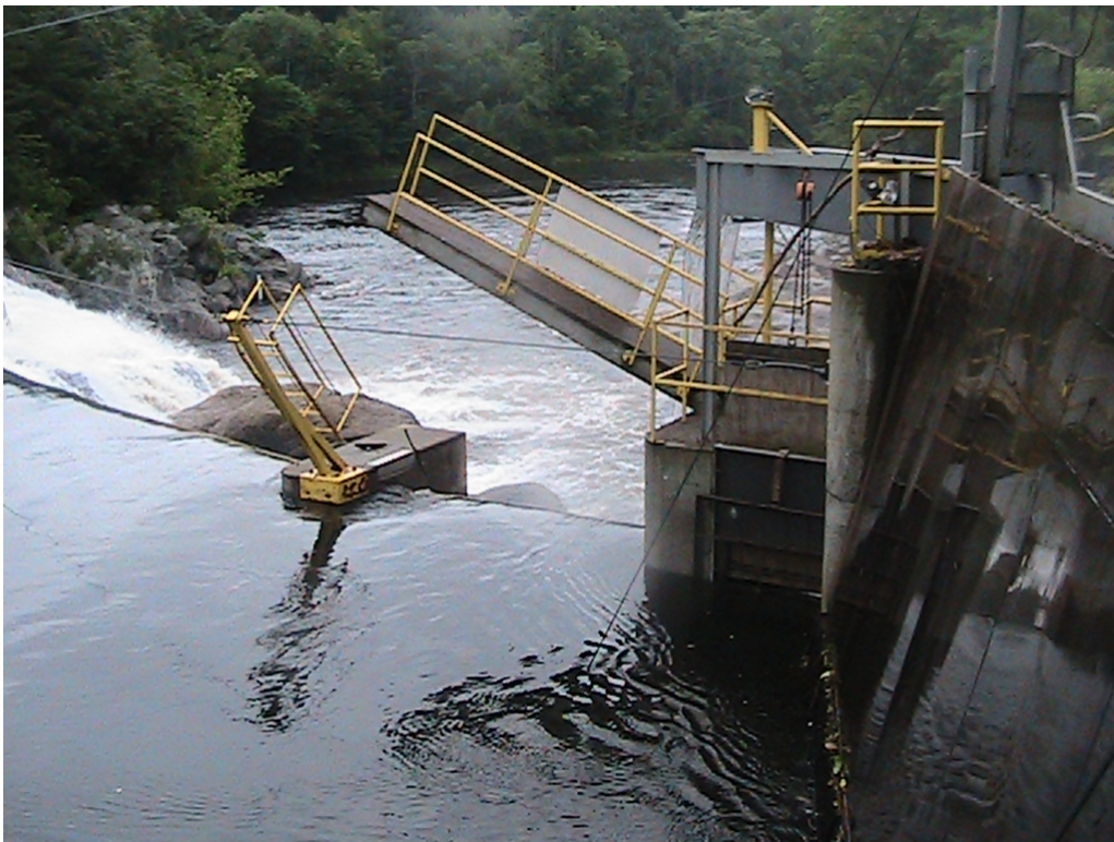
Photo 12D: Downstream Fish Passage Entrance and Trash Sluice
