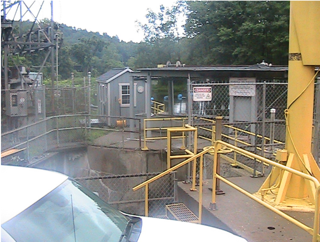
Photo 12E: Forebay and Intake Area (substation on left)
