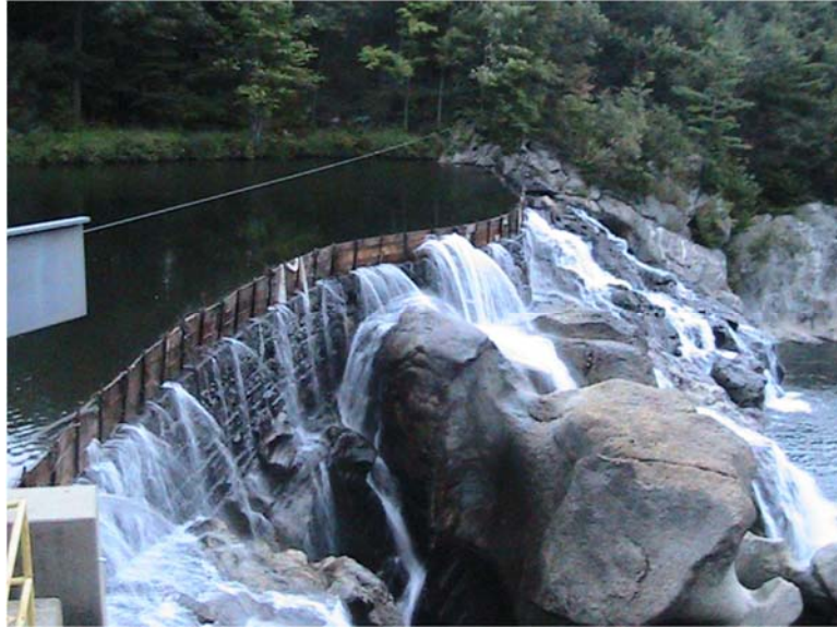
Figure 4 - Crescent Impoundment (facing West bank to East bank)
