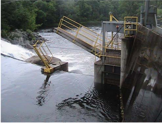
Figure 6 - Downstream Fish Bypass Entrance
