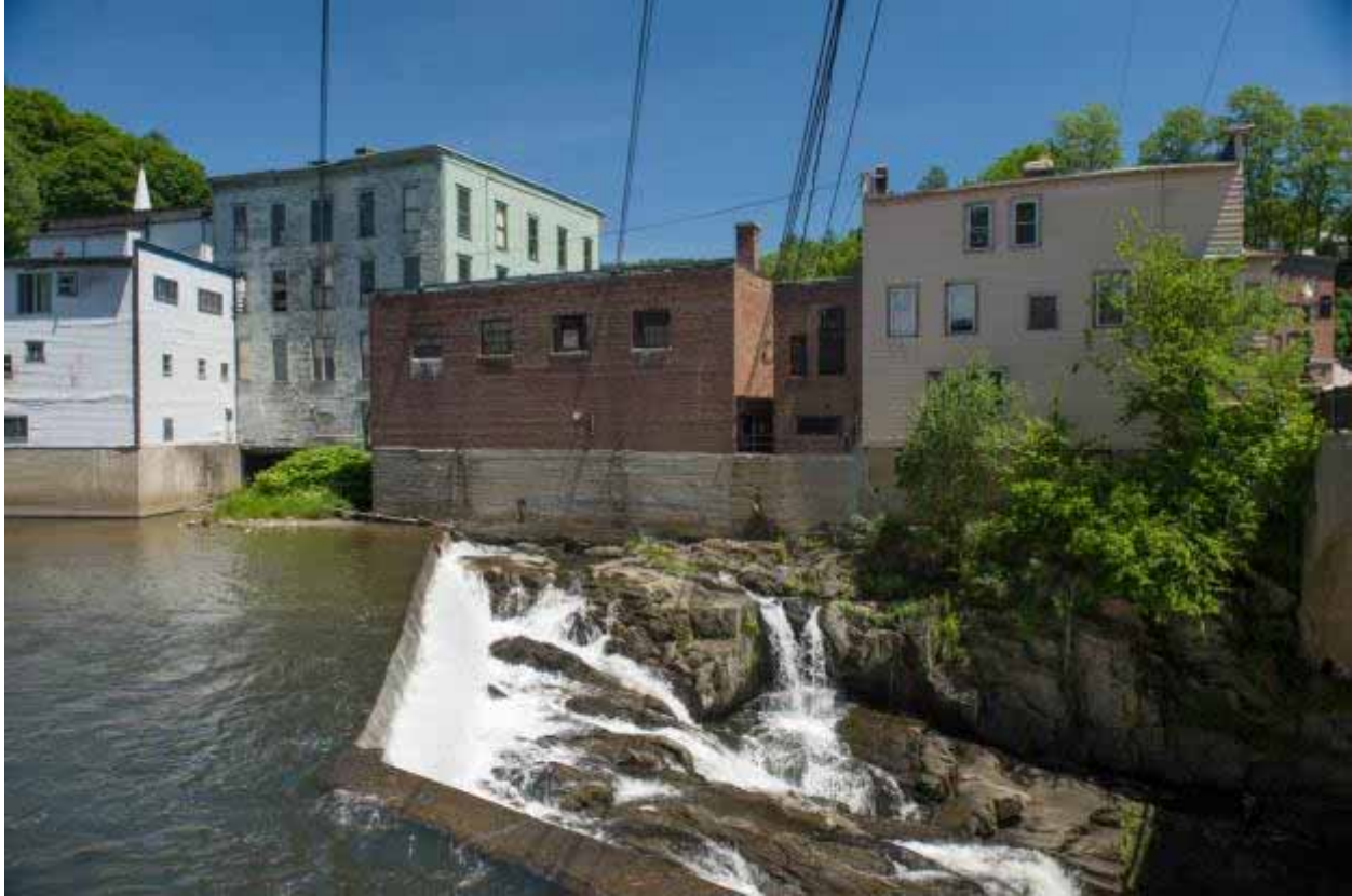
Figure 4 - Comtu Falls Impoundment looking across from powerhouse
