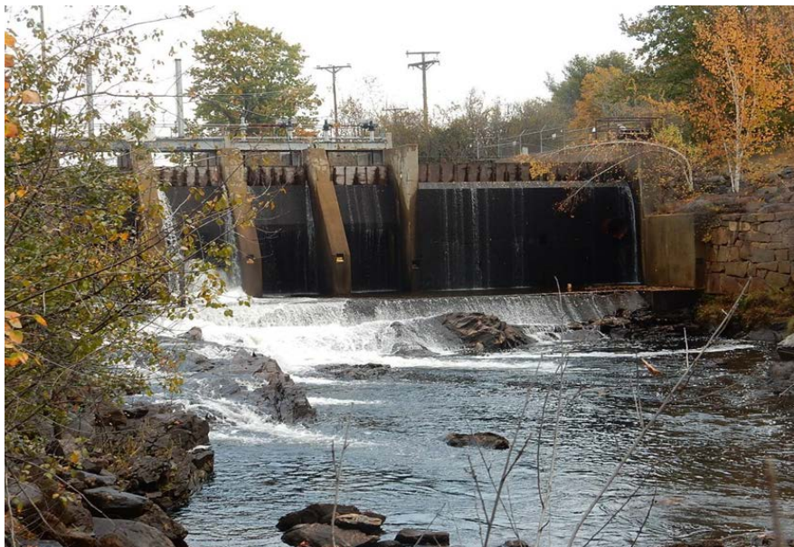
Figure 3 – Clement Project Dam and Spillway
