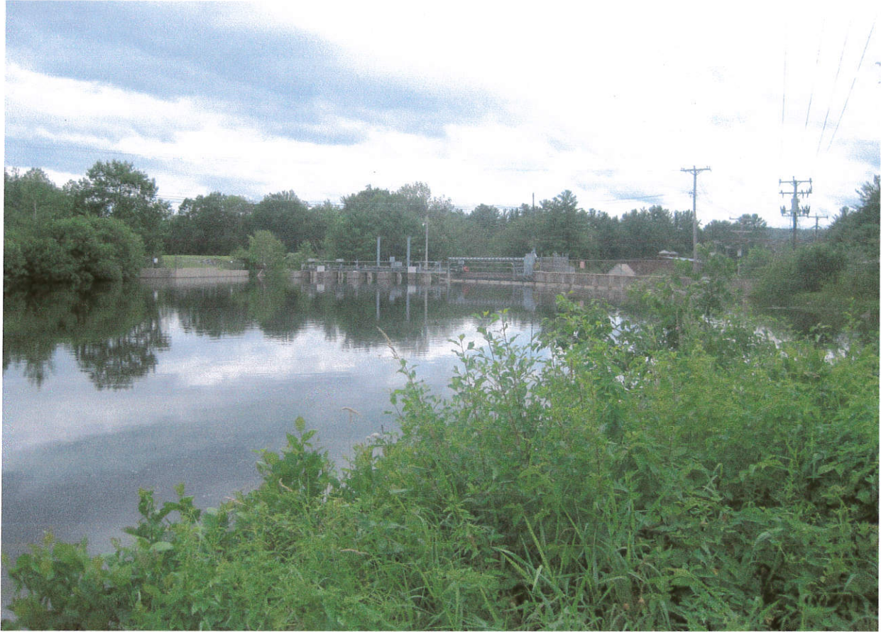
Clement Dam Impoundment
