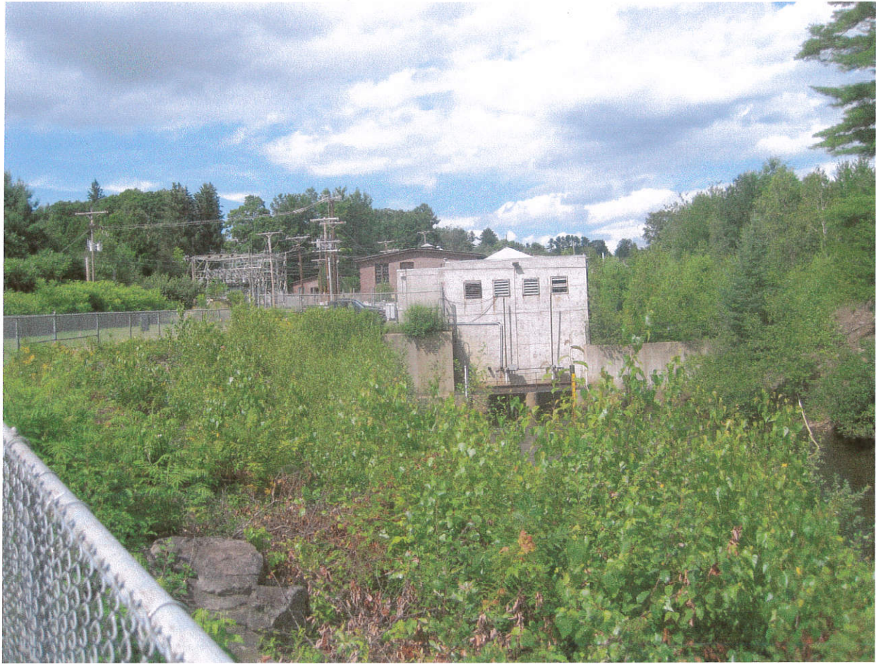
Clement Dam Powerhouse
