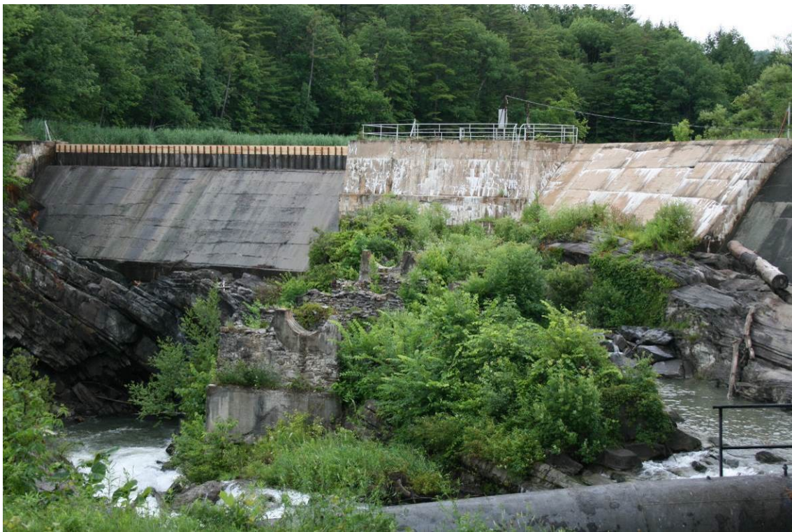
PHOTO 6 DAM SHOWING NEW FLASHBOARDS ON NORTH DAM WITH PENSTOCK IN FOREGROUND
