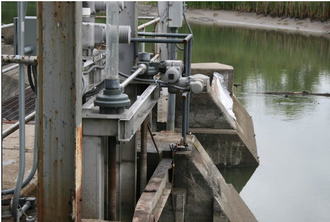
PHOTO 5 STAFF GAGE AT DAM (RESERVOIR DRAWN DOWN FOR FLASHBOARD INSTALLATION ON NORTH DAM)
