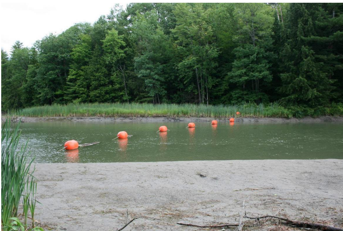
PHOTO 1 BOAT BARRIER (RESERVOIR DRAWN DOWN FOR FLASHBOARD INSTALLATION)
