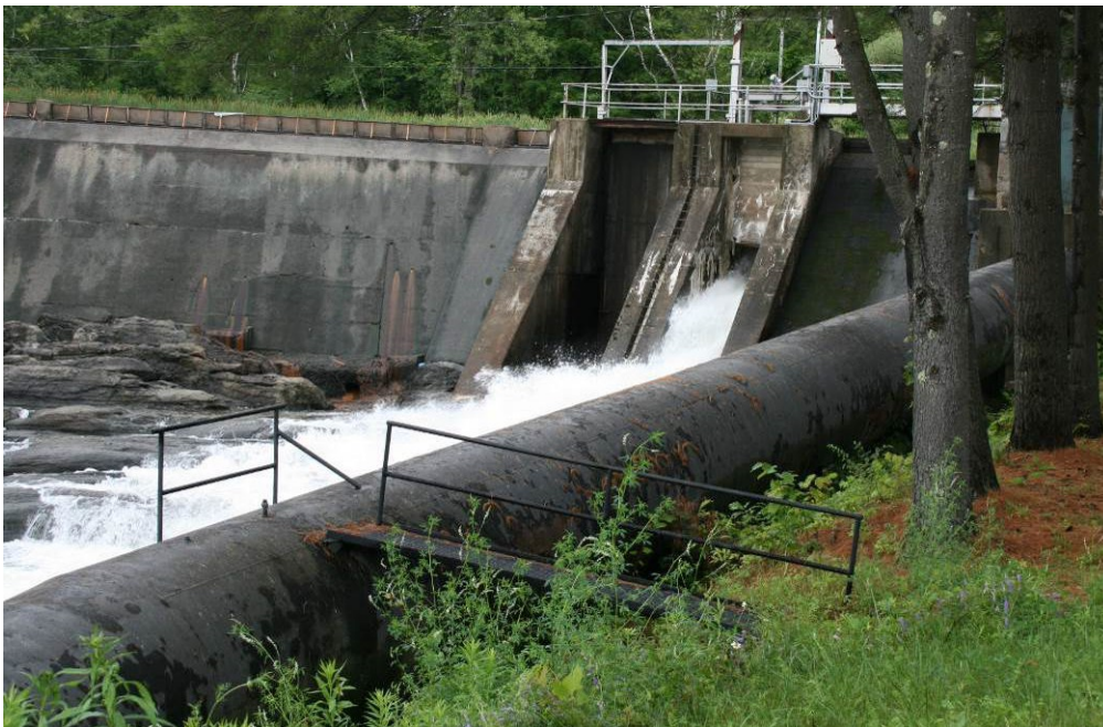
PHOTO 4 RELEASE FROM SOUTH DAM WITH PENSTOCK IN FOREGROUND
