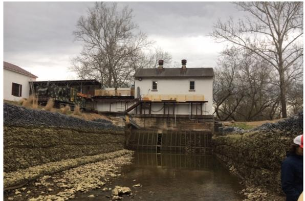
Figure 4- New Gabion Walls at Intake
