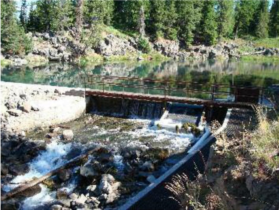
**Figure 5. View looking upstream at spillway with fishway in foreground along east (left) bank of river.**
