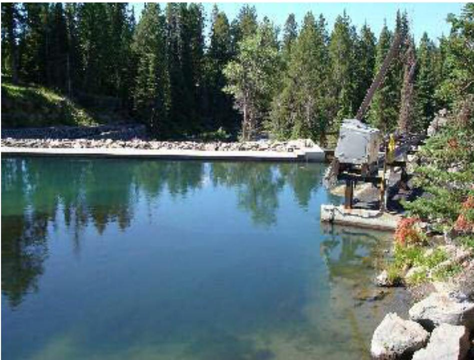
**Figure 6. View looking downstream with intake on right bank, automated trashrack rake visible.**
