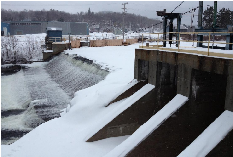
Figure 3. Side view of the dam's flood gates, spillway slab & timber crib spillway
