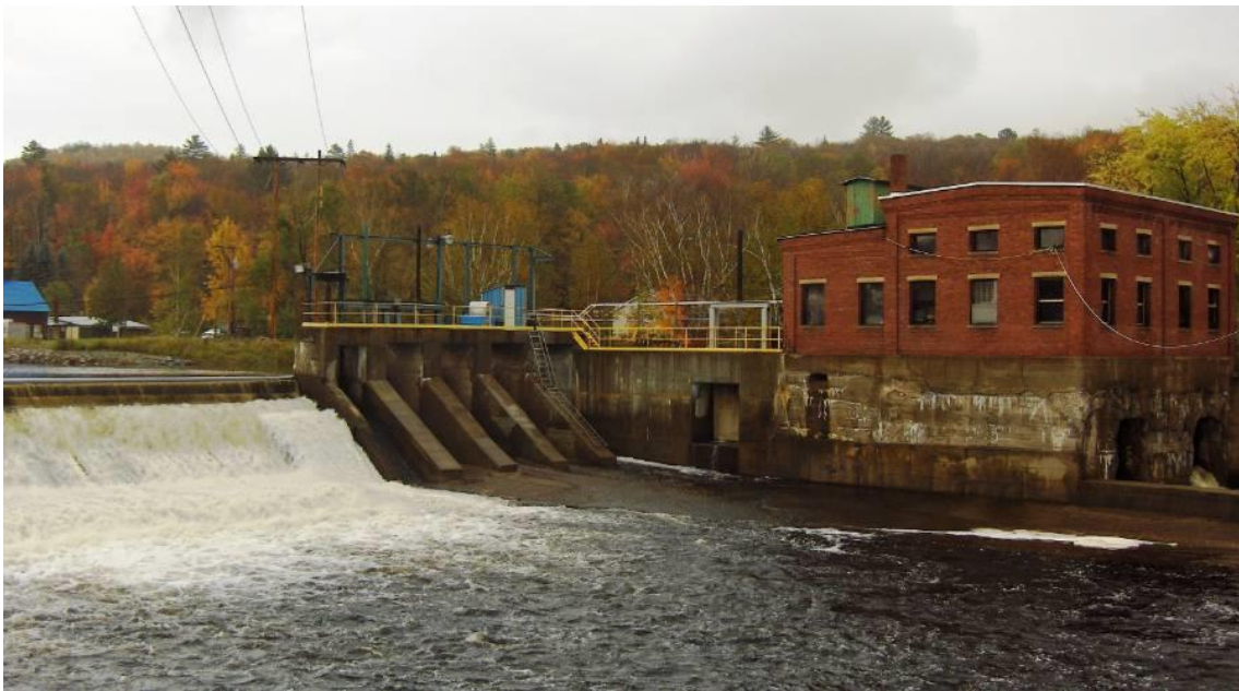
Figure 2. Overview of the Brooklyn Dam, including powerhouse, spillway slab, flood gates & timber crib spillway
