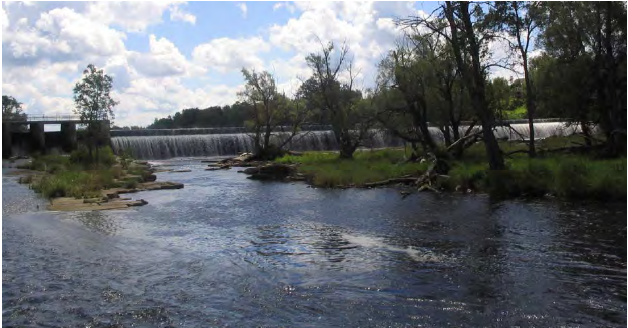
Deferiet dam with 3-foot pneumatic flashboards
