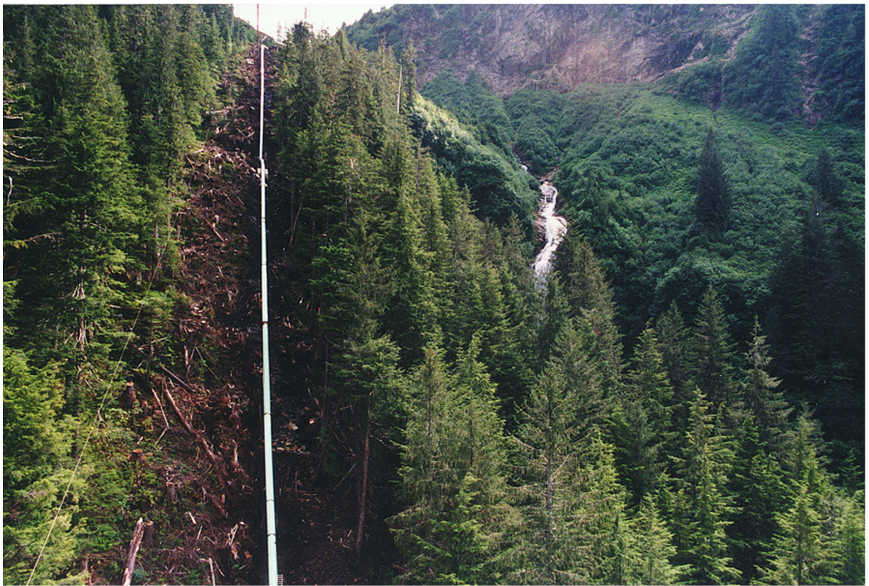
PENSTOCK COMING DOWN SLOPE FROM LAKE WITH OUTLET STREAM AT RIGHT
