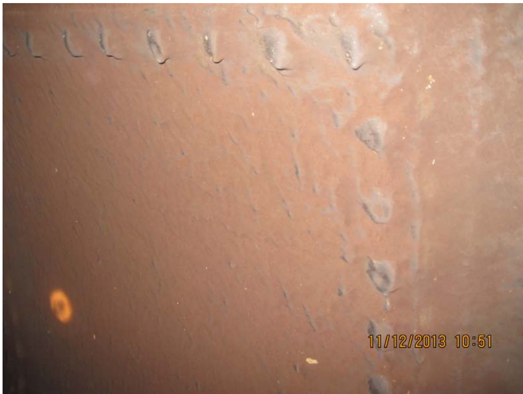
PHOTO 24 – PENSTOCK NO. 3 COATED RIVET JOINTS (1)
