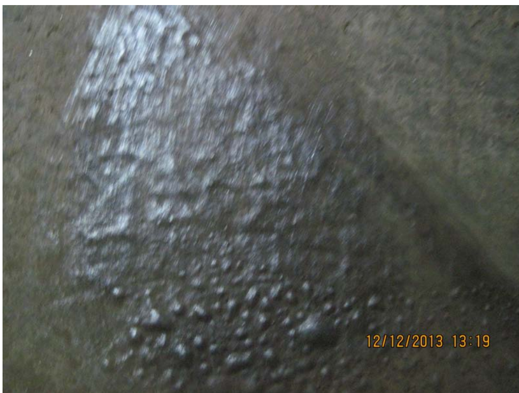
PHOTO 14 – PENSTOCK NO. 2 IRREGULAR SURFACE OF INTERIOR COATING
