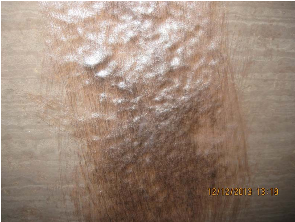
PHOTO 15 – PENSTOCK NO. 2 SCRAPED SURFACE OF INTERIOR COATING TO OBTAIN THICKNESS READINGS
