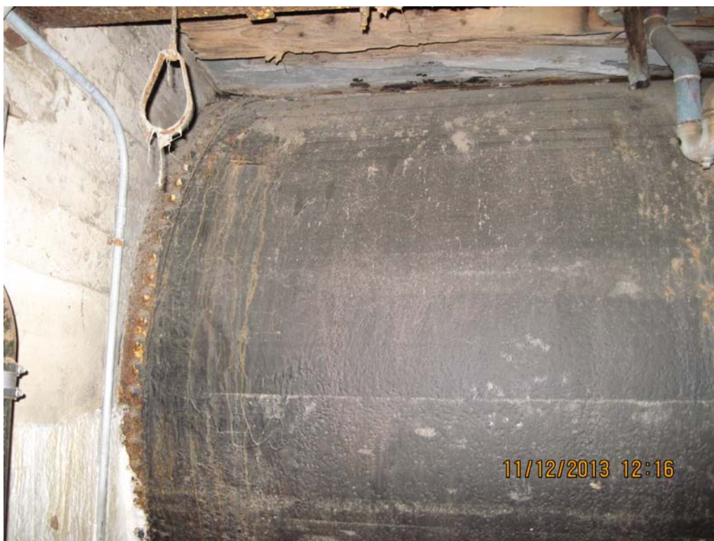
PHOTO 37 – PENSTOCK NO. 4 PAINTED SECTION OF EXPOSED LEFT FACE
