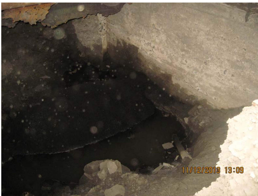
PHOTO 4 – DISPLACED SOIL BELOW PENSTOCK NO. 2 FAILURE
