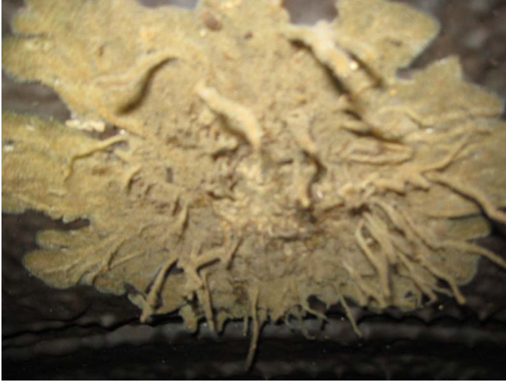
PHOTO 35 – BACTERIA ATTACHED TO INTERIOR PENSTOCK COATING (MULTIPLE LOCATIONS)
