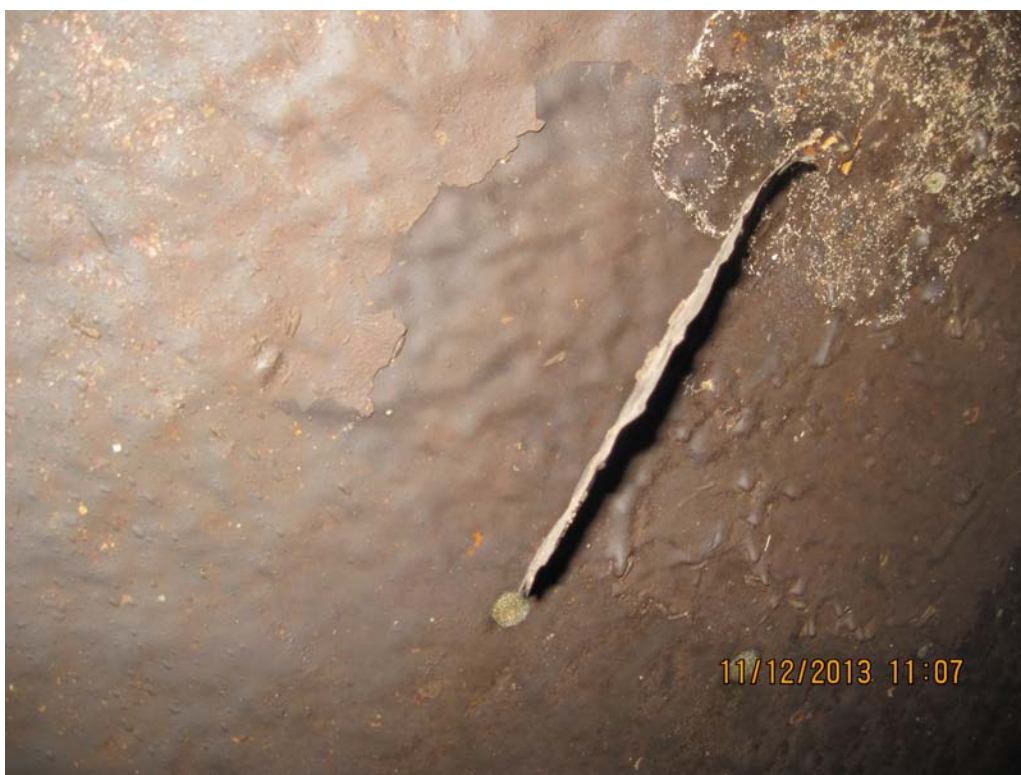
PHOTO 20 – DELAMINATION OF PENSTOCK NO. 3 INTERIOR (2)
