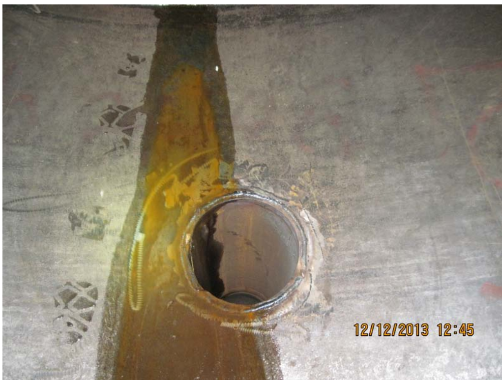
PHOTO 11 – PENSTOCK NO. 2 NEW FLOOR DRAIN AT NEW SECTION
