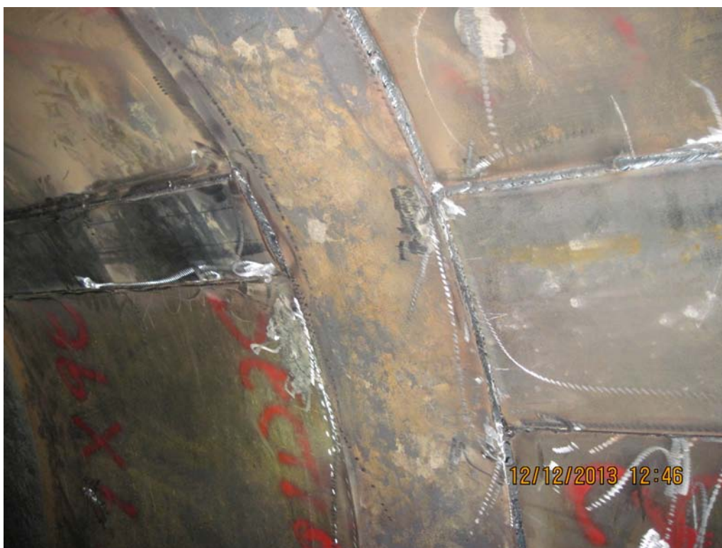
PHOTO 8 – PENSTOCK NO. 2 LONGITUDINAL AND CIRCUMFERENTIAL JOINTS OF REPAIRED SECTION (2)
