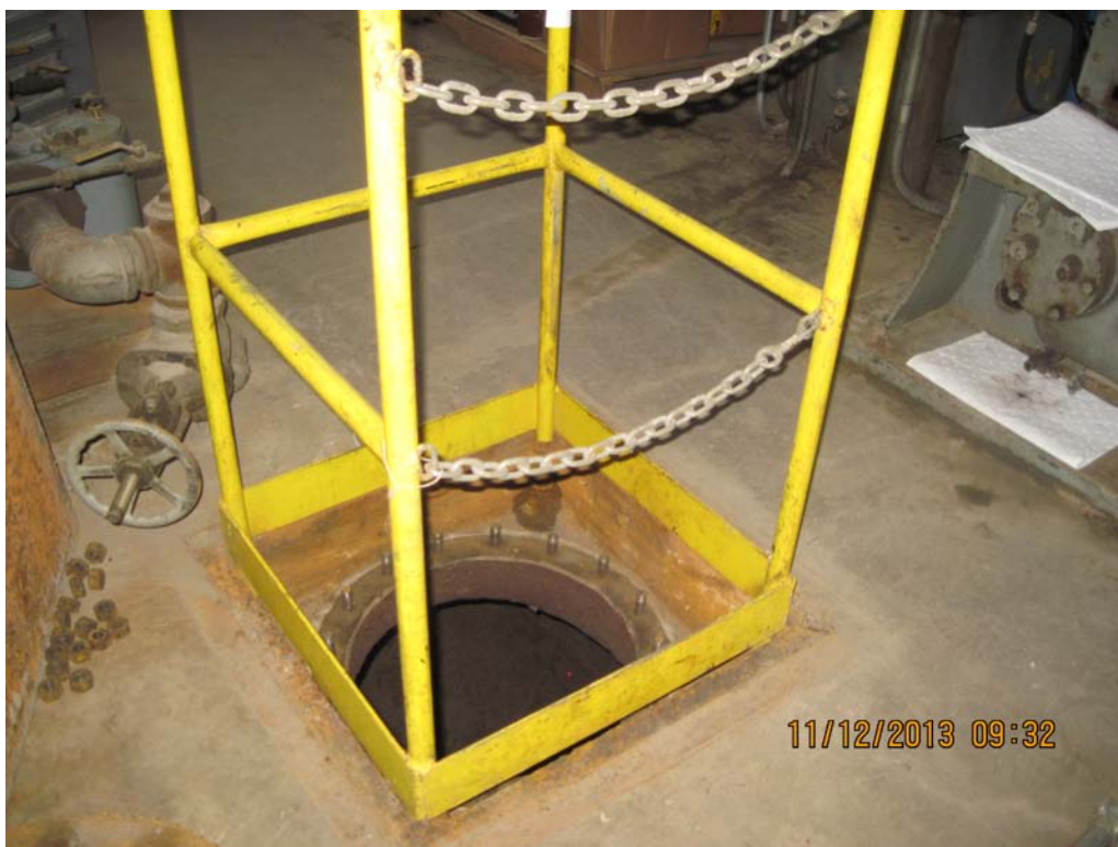
PHOTO 5 – MANHOLE ENTRANCE TO PENSTOCK IN POWERHOUSE
