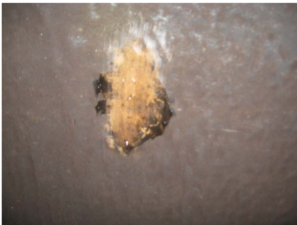
PHOTO 28 – CLEANED INTERIOR SURFACE OF PENSTOCK FOR THICKNESS MEASUREMENTS (1)
