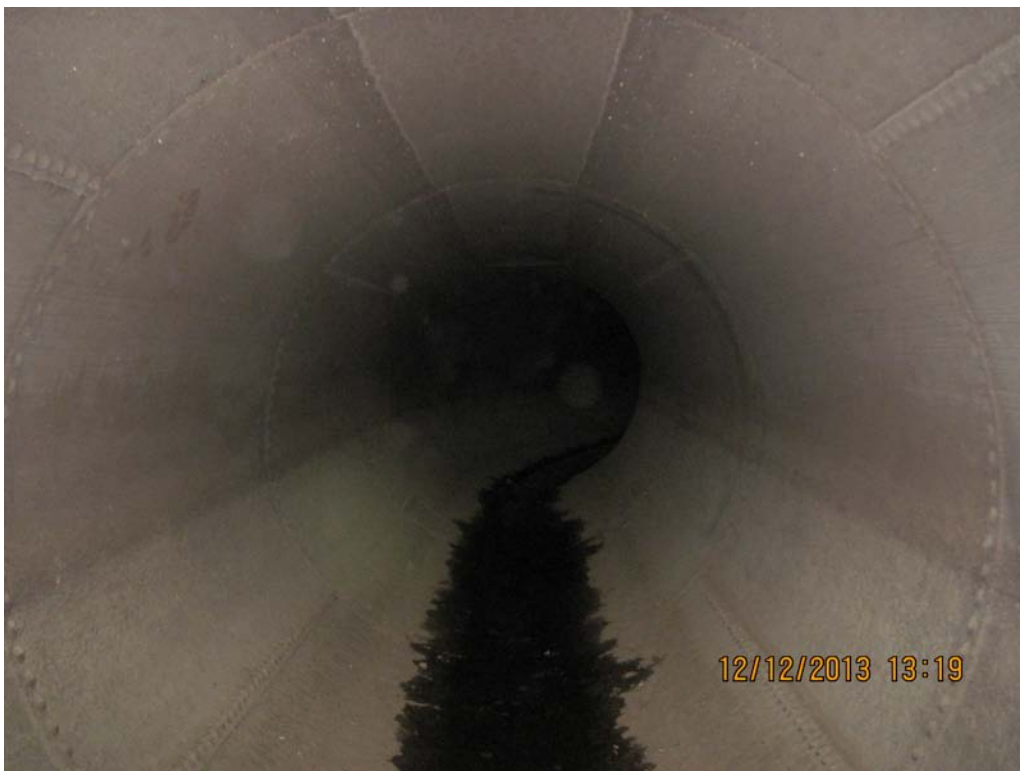
PHOTO 16 – PENSTOCK NO. 2 INTERIOR COATED SECTION & WATER LINE
