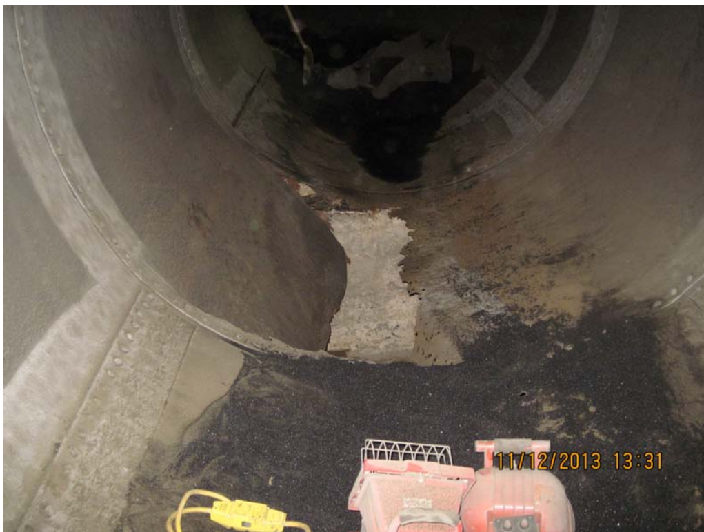
PHOTO 1 – INTERIOR OF PENSTOCK NO. 2 FAILURE LOOKING UPSTREAM
