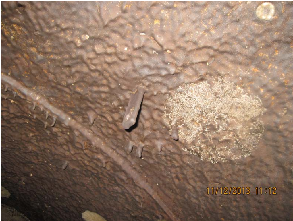
PHOTO 33 – PATCH LOCATION IN PENSTOCK NO. 4
