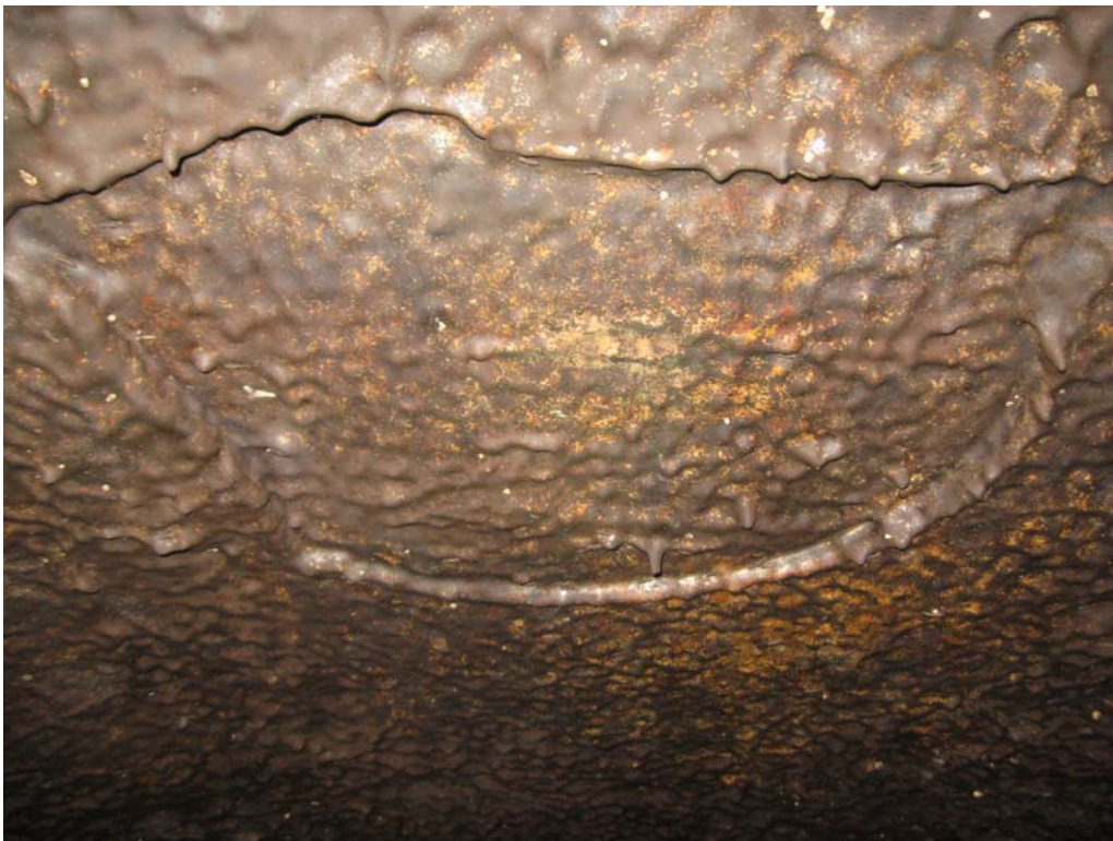
PHOTO 32 – PENSTOCK NO. 4 DELAMINATED COATING
