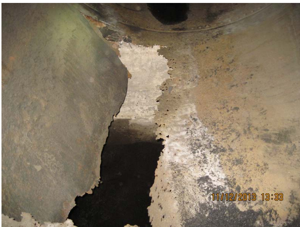
PHOTO 2 – CLOSER VIEW OF PENSTOCK NO. 2 FAILURE
