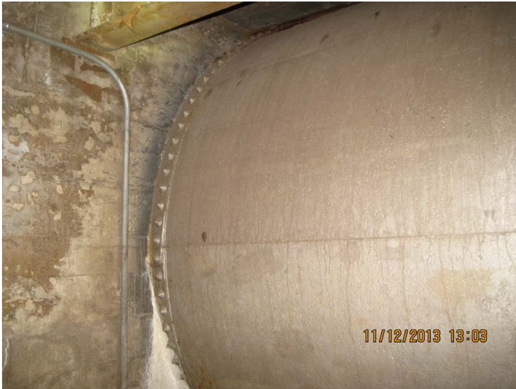
PHOTO 31 – PENSTOCK NO. 3 EXPOSED & PAINTED DOWNSTREAM LEFT FACE
