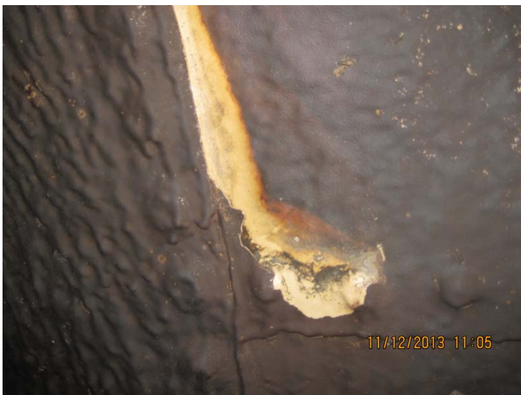
PHOTO 18 – DELAMINATION OF PENSTOCK No. 3 COATING
