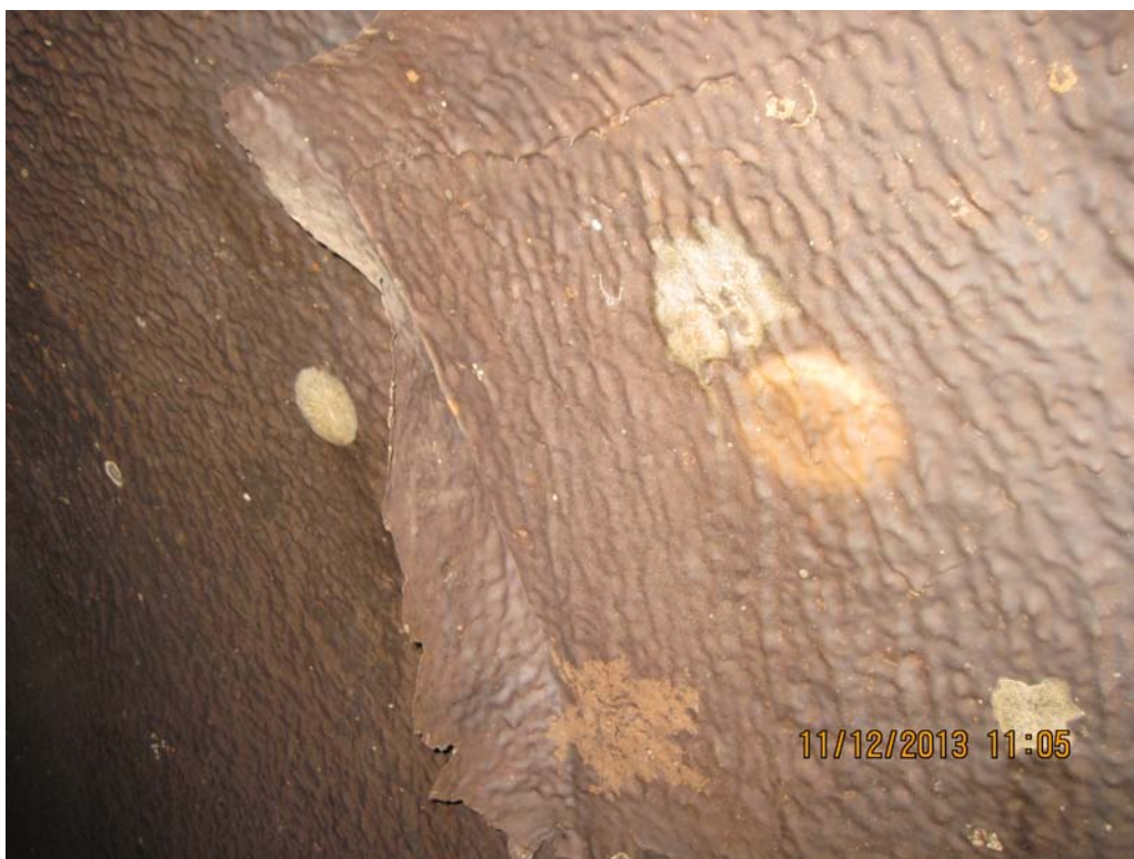
PHOTO 19 – DELAMINATION OF PENSTOCK NO. 3 INTERIOR (1)
