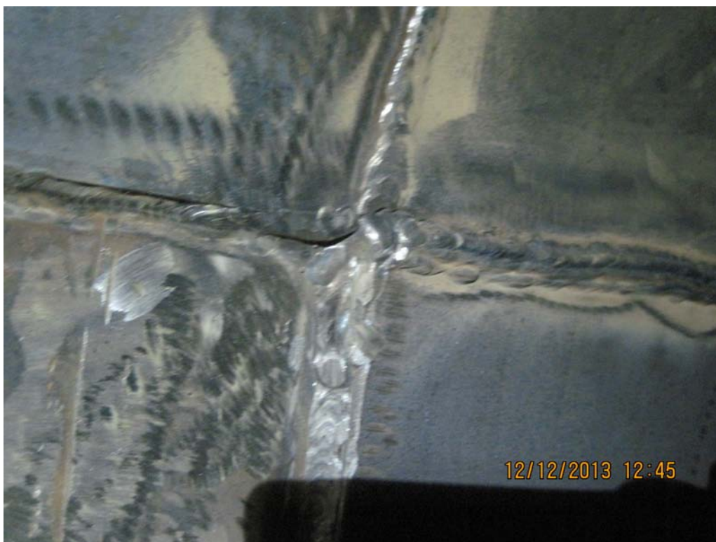
PHOTO 9 – PENSTOCK NO. 2 CLOSE UP OF 1/4 INCH FILLET WELDS
