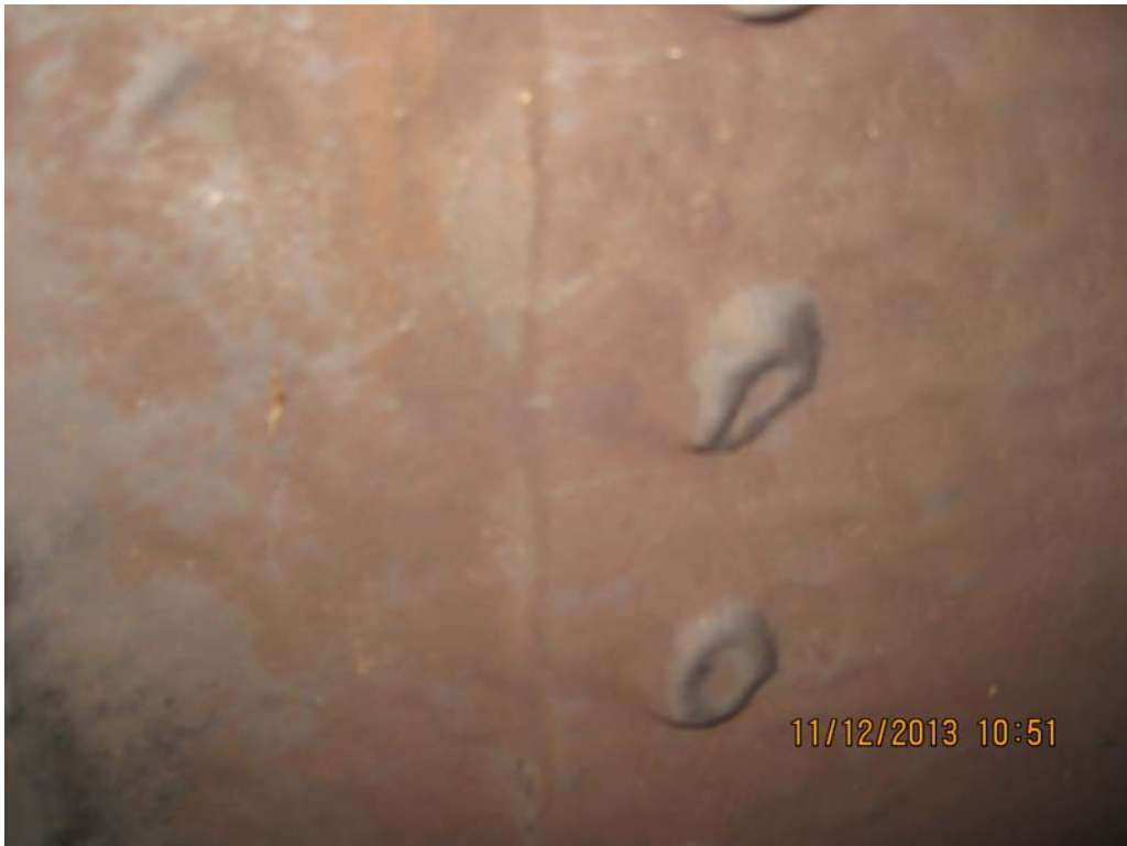
PHOTO 26 – PENSTOCK NO. 3 CLOSE UP OF COATED RIVER JOINTS
