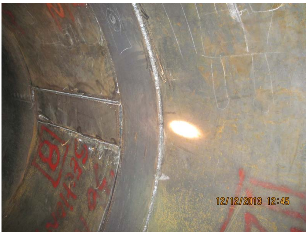
PHOTO 7 – PENSTOCK NO. 2 LONGITUDINAL AND CIRCUMFERENTIAL JOINTS OF REPAIRED SECTION (1)
