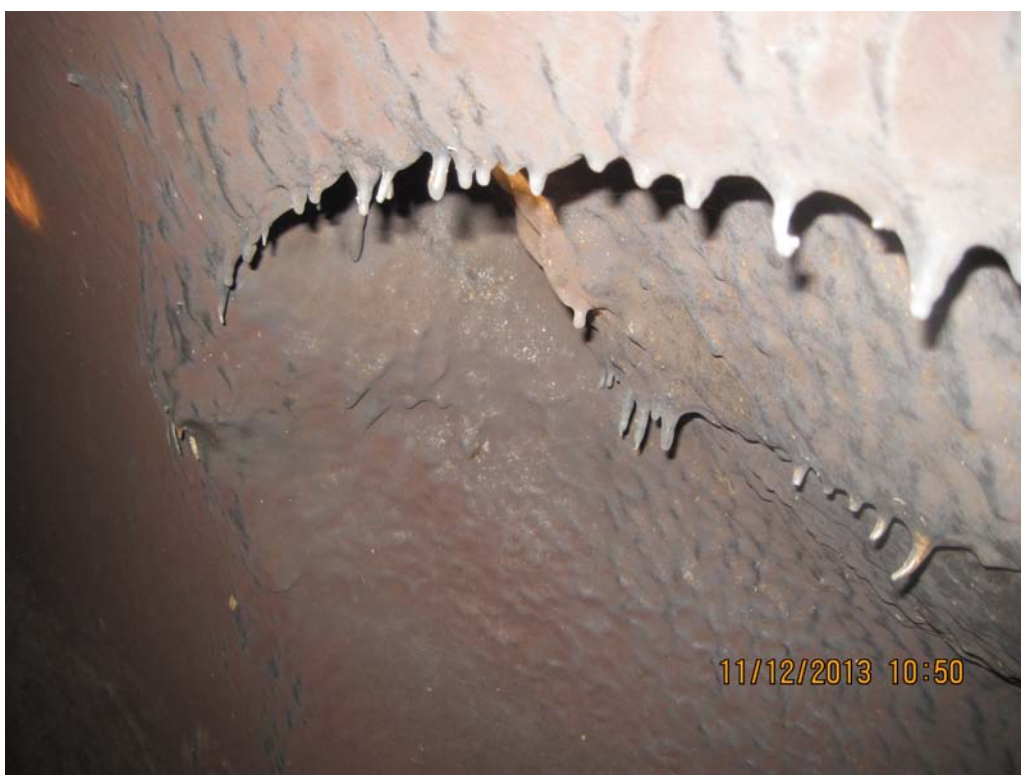
PHOTO 17 – OVERCOATED PENSTOCK No. 3 INTERIOR
