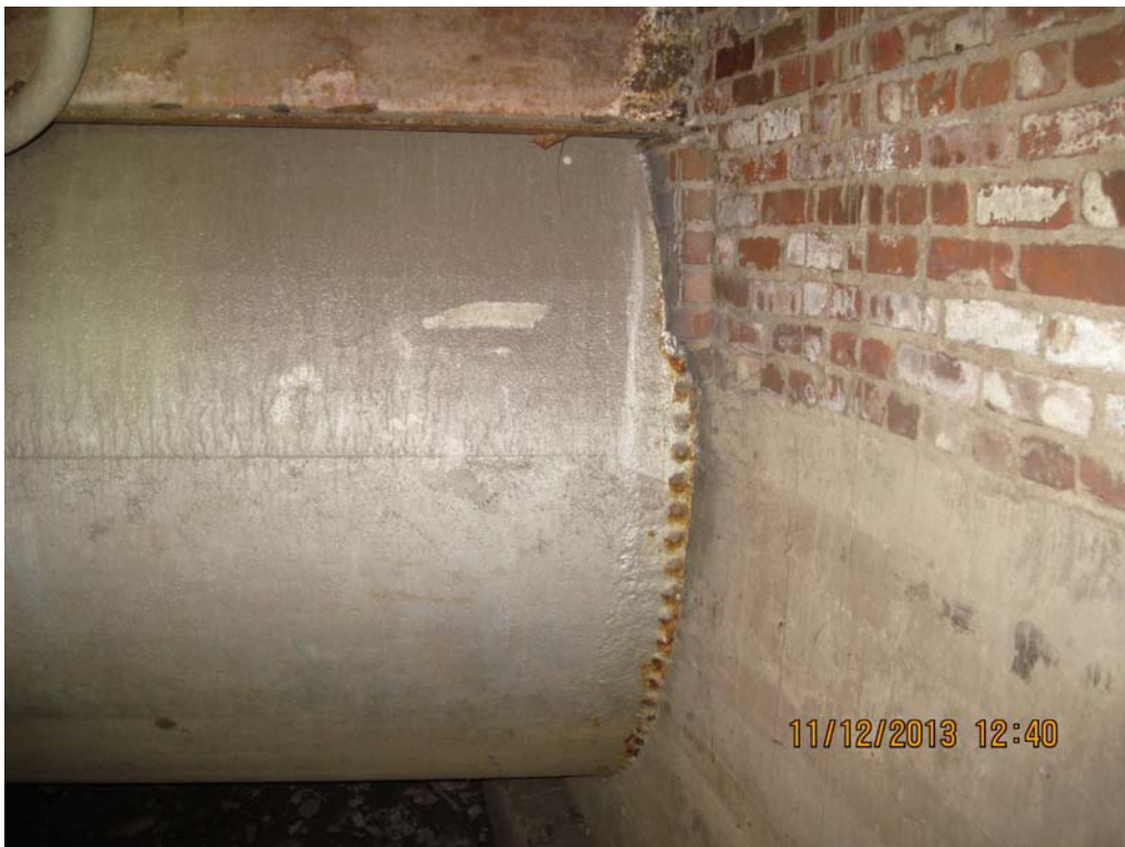
PHOTO 30 – PENSTOCK NO. 3 EXPOSED & PAINTED UPSTREAM LEFT FACE
