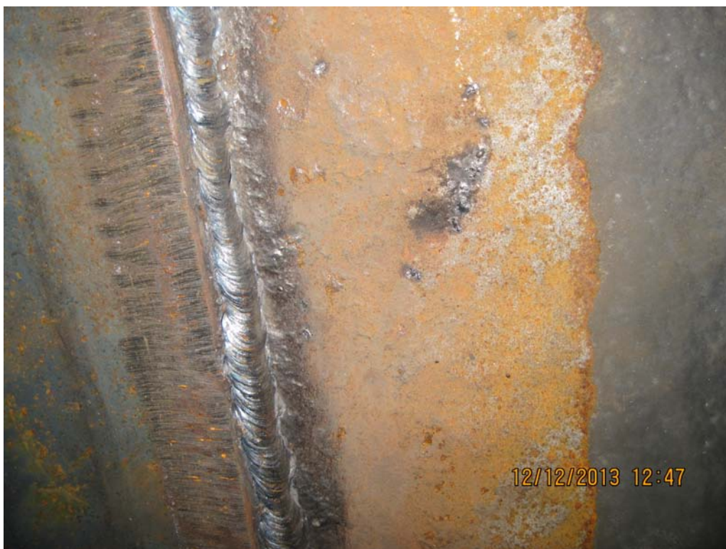
PHOTO 10 – PENSTOCK NO. 2 CLOSE UP OF 1/4 INCH FILLET WELD & SAND BLASTED COATING
