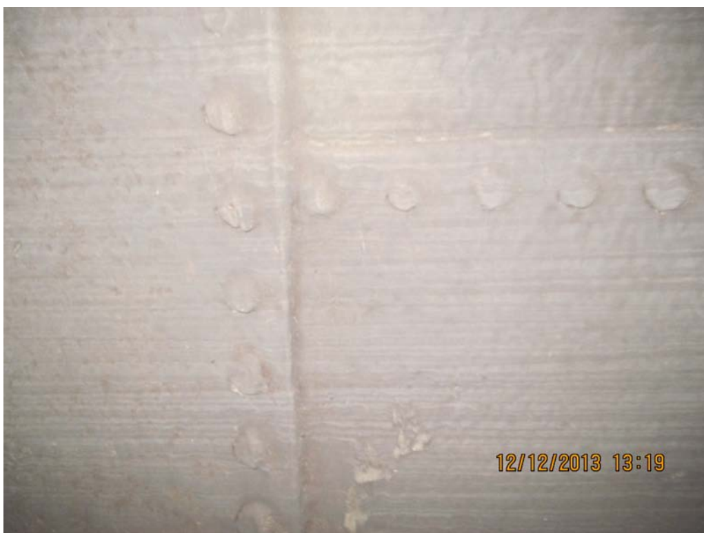
PHOTO 12– PENSTOCK NO. 2 INTERIOR COATING & RIVETED LAP SEAMS
