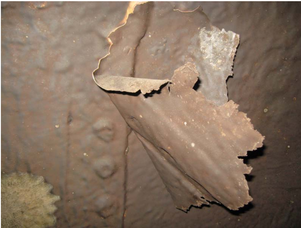
PHOTO 21 – DELAMINATION OF PENSTOCK NO. 3 INTERIOR (3)
