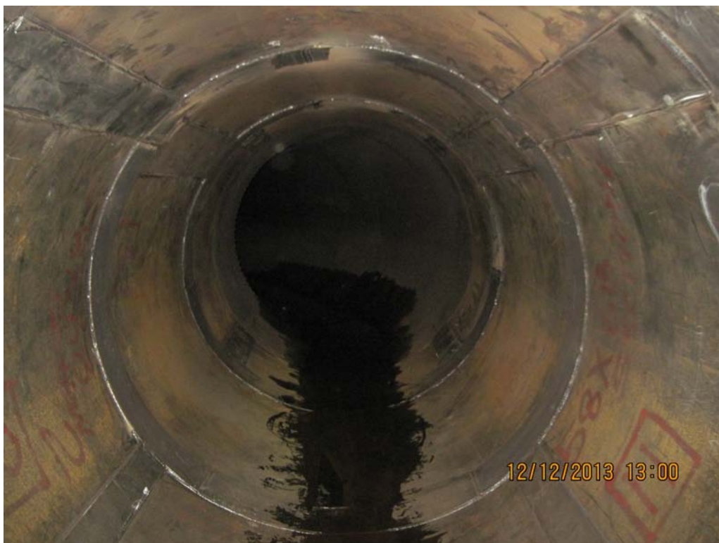
PHOTO 6 – PENSTOCK NO. 2 INTERIOR STEEL SLEEVE REPAIRED SECTION
