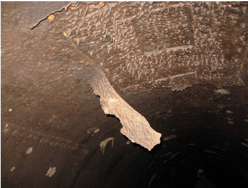
PHOTO 34 – PENSTOCK NO. 4 PATCH PLATE (APPROX. 2' X 4') AT STATION 0+86
