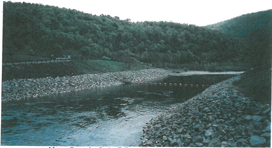
Matson Generating Station Tailrace (Flow Approximately 500 cfs).
