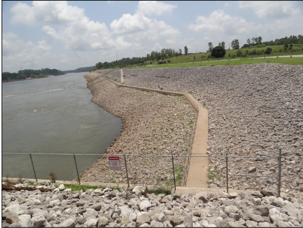
Photo 5. View looking downstream from the powerhouse access road at the tailrace fishing access ramp and walkway. The project boundary follows the top of the riprapped area.
