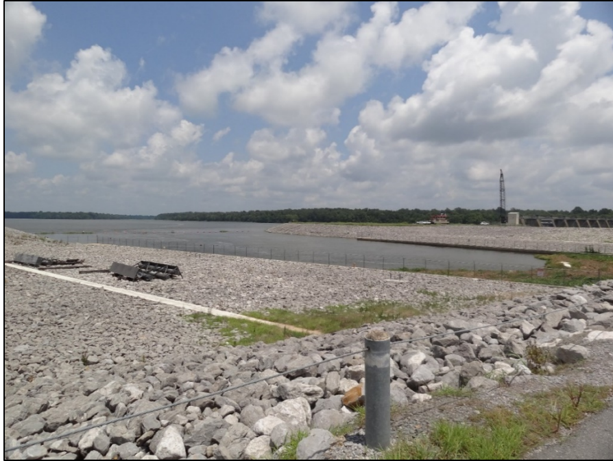
Photo 3. View across headrace channel toward the dam and spillway at far right. Boat barrier (background) at inlet to the headrace channel. Vegetation in headrace (far right) is water hyacinth that floated downstream from coves upstream of the dam.
