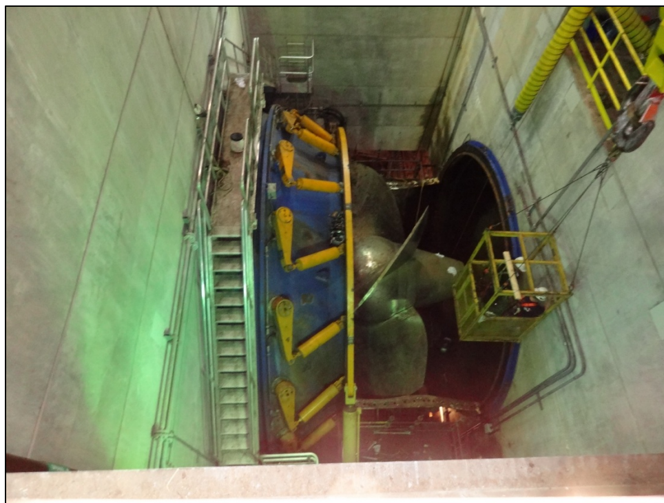
Photo 10. View inside of powerhouse showing Unit No. 2 undergoing rehabilitation.
