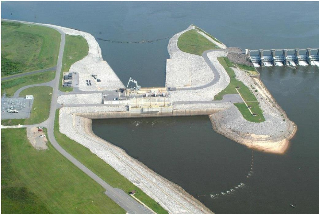
The powerhouse contains three horizontal-shaft, bulb-type, axial-flow hydraulic turbine-generator units. Each of the turbines is of the Kaplan propeller type with four adjustable blades, and adjustable wicket gates, complete with an electronically controlled hydraulically operated governor. The maximum net power head available to the turbines is approximately 44.5 feet. The turbines operate under a net head which normally ranges from 5 feet to 37 feet. The turbines
