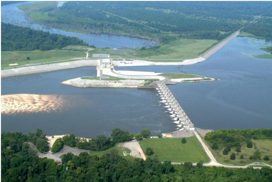
*Aerial view looking west at Arkansas River Dam No. 2. The hydroelectric project, built into an existing non-overflow embankment, is to the west of the Corps spillway visible in foreground. The water body visible in the upper left of the photo is the old Arkansas River channel, cut off at the time Corps constructed the dam in the late 1960s, and fed by a water supply pipeline from the dam. See text for additional information.*
