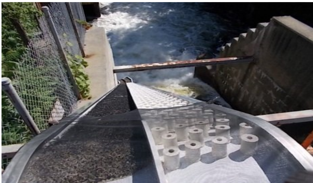
Eel Ladder looking down from spillway deck
