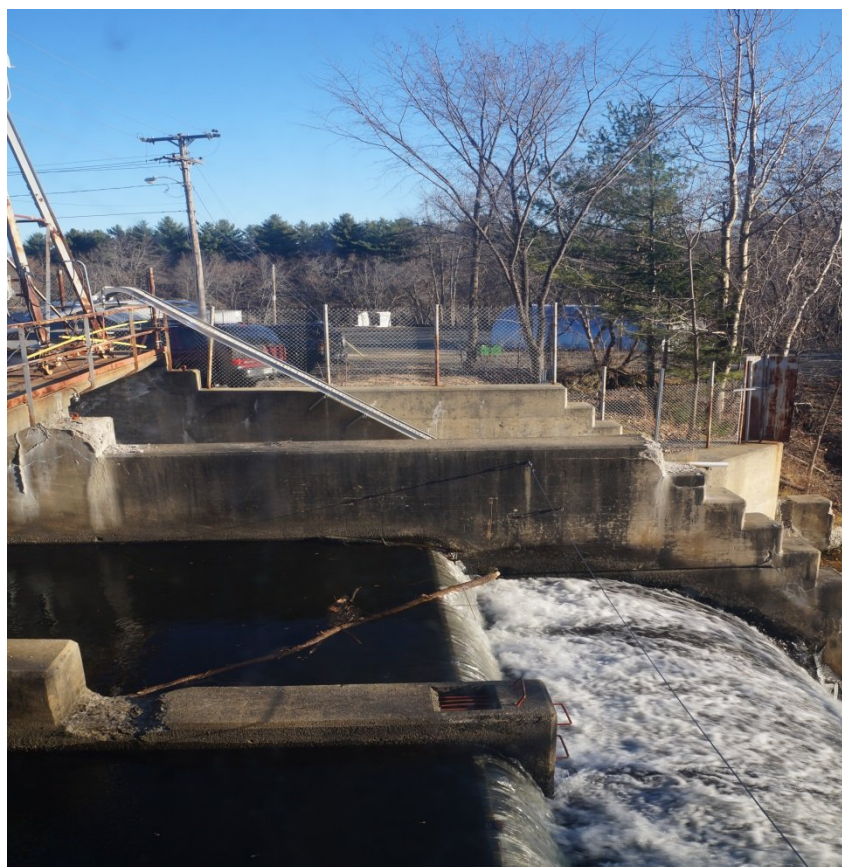
Eel Ladder in background extending down from spillway deck
