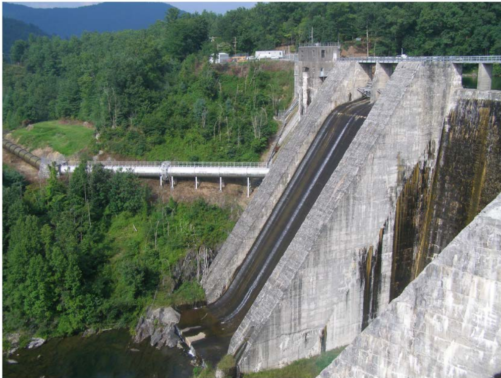
Santeeetlah Right Thrust Block and Spillway
