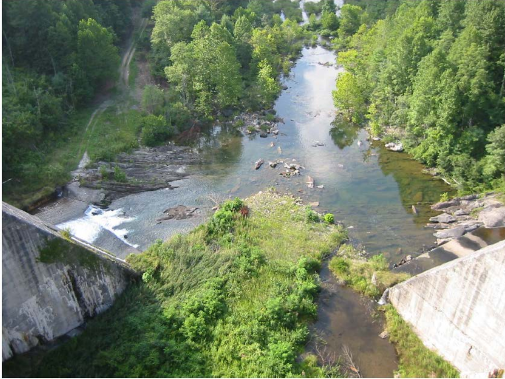
Santeetlah Plunge Pool and Bypass Reach
