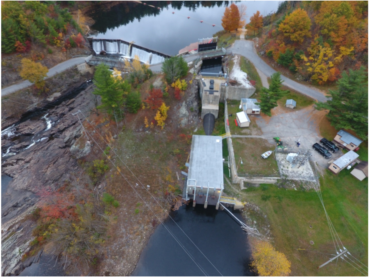
PHOTO 4 VIEW OF PENSTOCK AND POWERHOUSE
