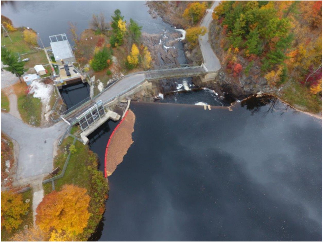
PHOTO 2 EMERYVILLE PROJECT LOOKING DOWNSTREAM
