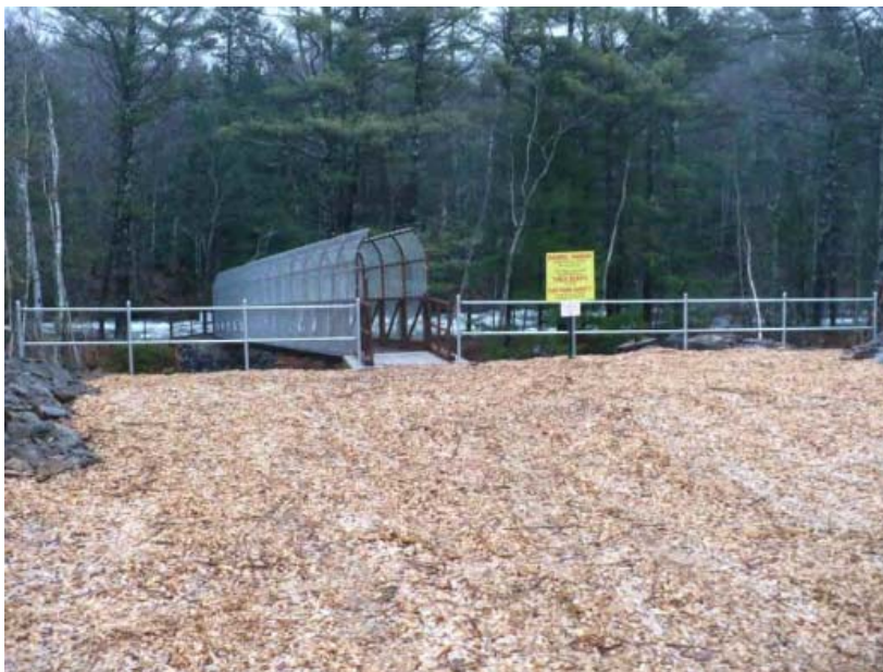
Figure 2. Pedestrian bridge entrance
