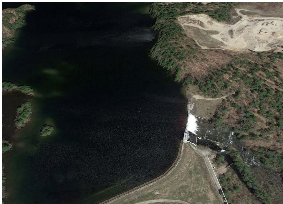
Satellite image of the lower impoundment at the Dundee Project (FERC No. P-2942).
