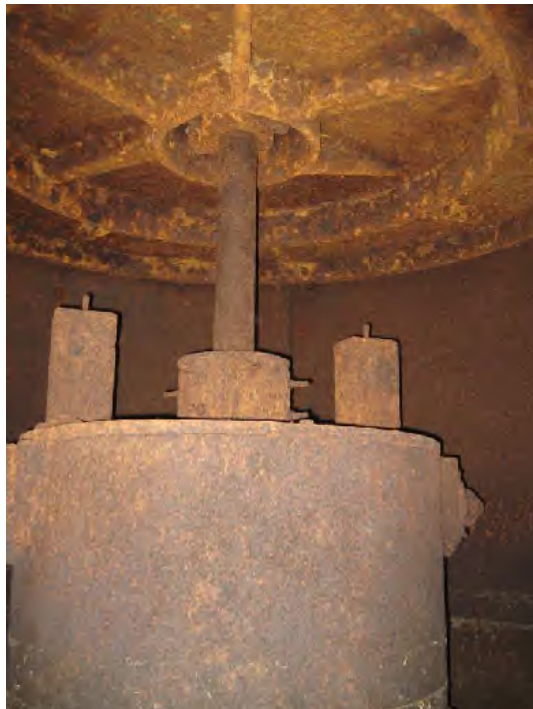
Photo 4 Turbine Within Pressure Case
