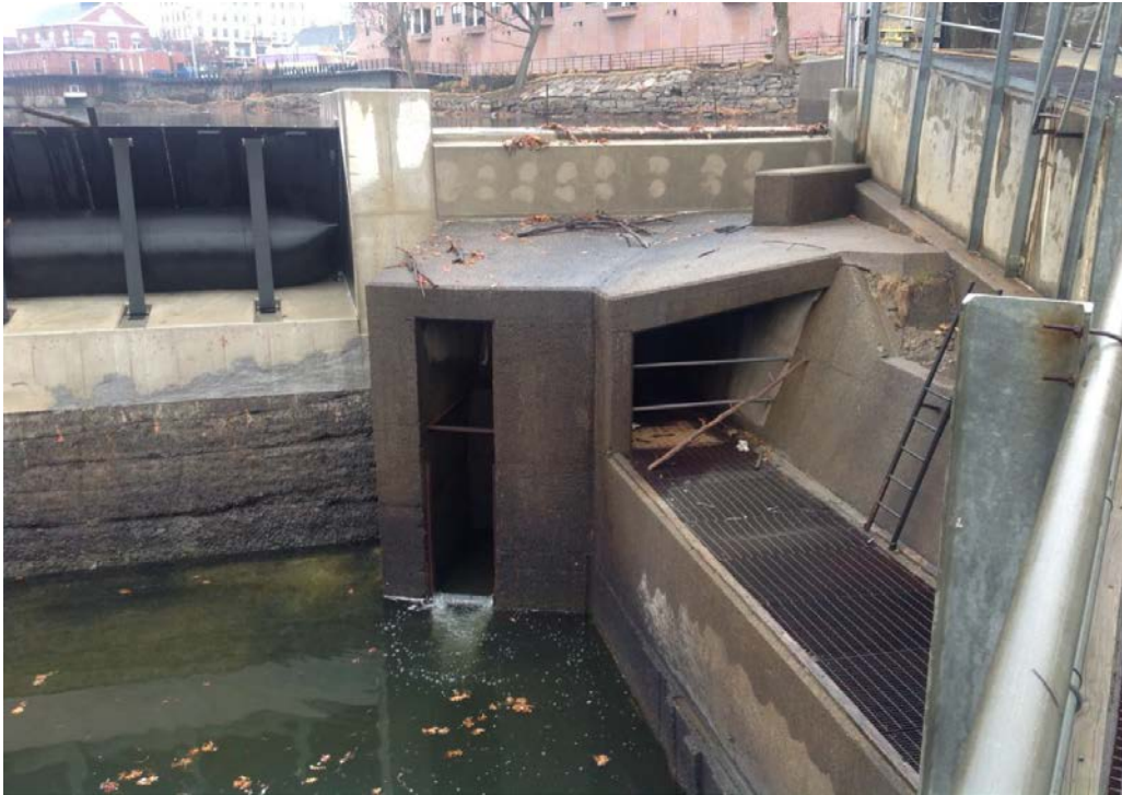
Figure 4 - 38 Foot Section of Spillway Above Upstream Fish Passage
