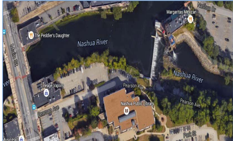
Figure 2 - Jackson Mills Dam
