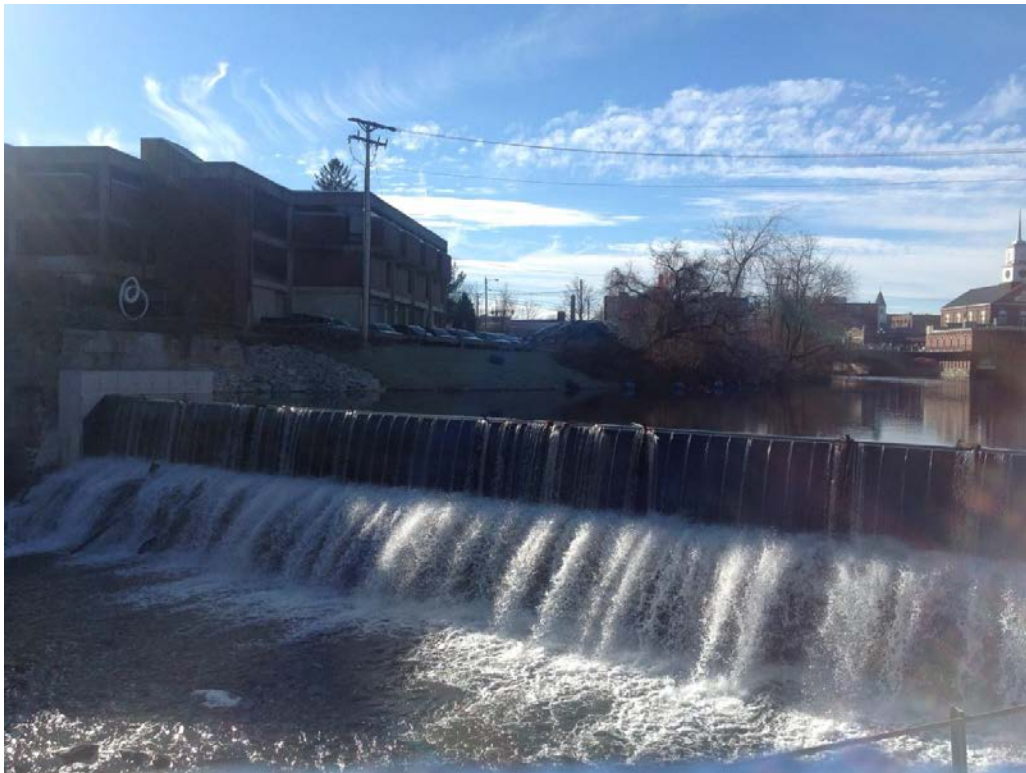
Figure 3 - Pneumatic Crest Gates – Looking Upstream
