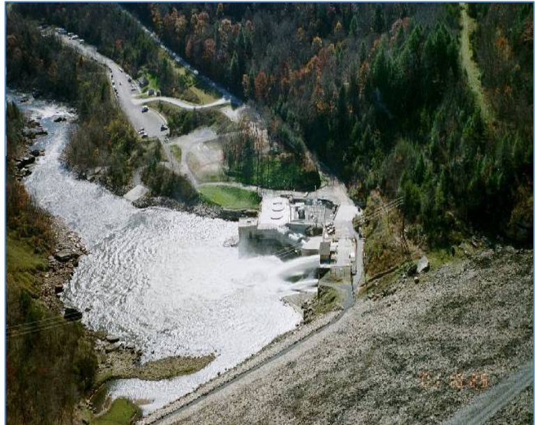
Figure 2 - View of Corps Valve House from Dam
