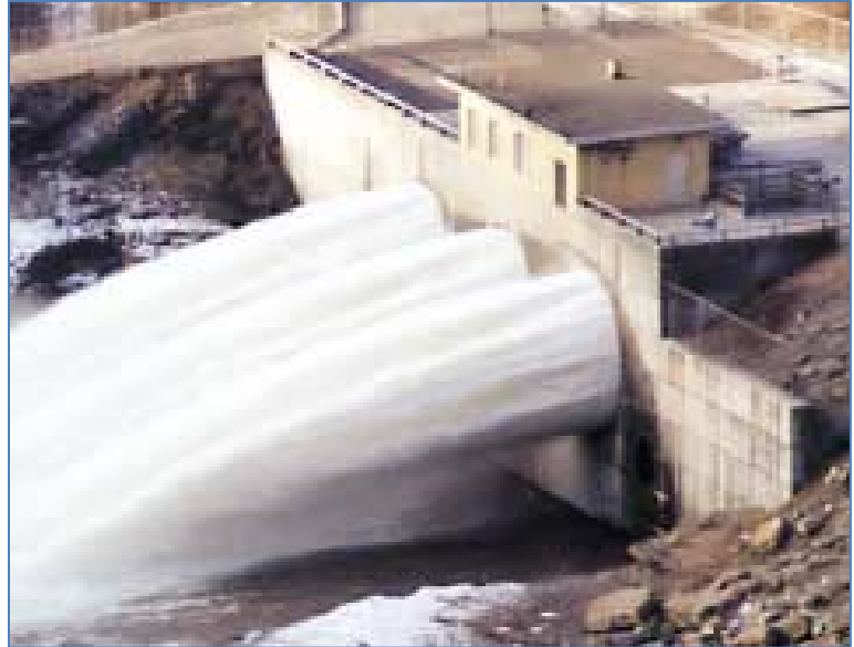
Figure 3 - View of Howell-Bunger Valves
