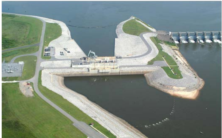
Figure 3 - Power View Looking Upstream
