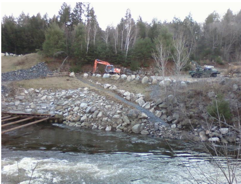
Figure 1 - Canoe Portage Trail completed at Ashuelot
