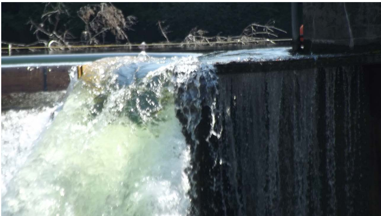
PHOTO 5 VIEW OF THE DOWNSTREAM FISH PASSAGE FACILITY ADJACENT TO THE INTAKE. THE DOWNSTREAM FISHWAY PROVIDES THE 88 CFS MINIMUM FLOW RELEASE YEAR-ROUND.
