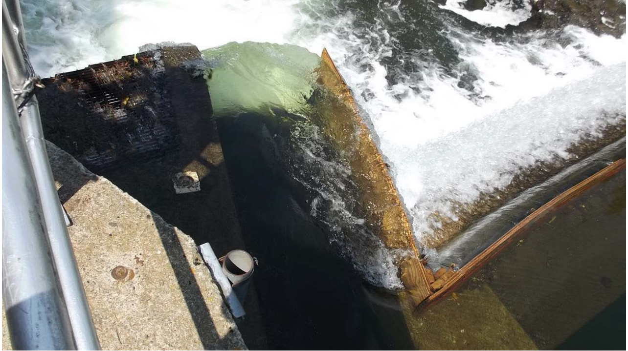
PHOTO 6 VIEW OF THE DOWNSTREAM FISH PASSAGE FACILITY AS SEEN FROM THE DECK OF THE INTAKE STRUCTURE
