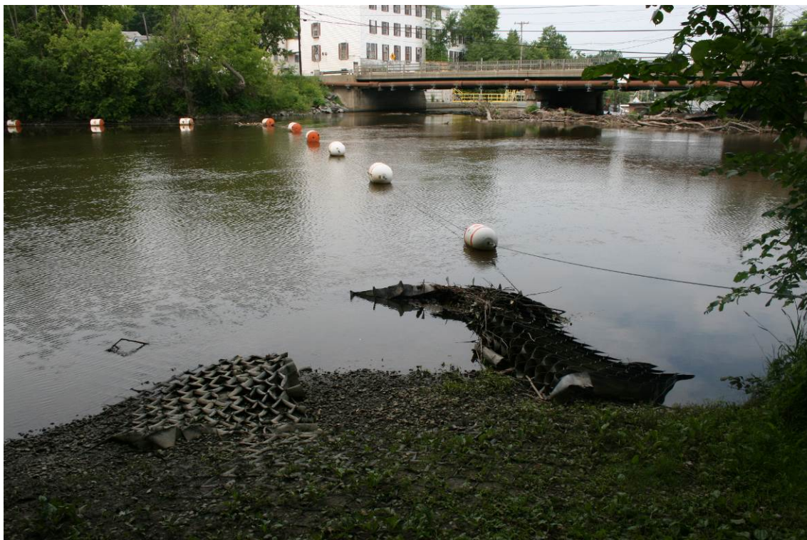
Photo 7. Canoe take-out, boat ramp with damaged geotextile mat and boat barrier in the background.
