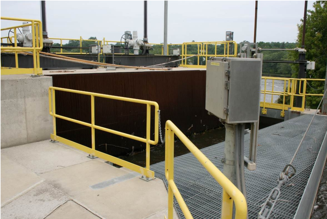
Photo 3. New headgates, intake, screen and monitoring equipment.
