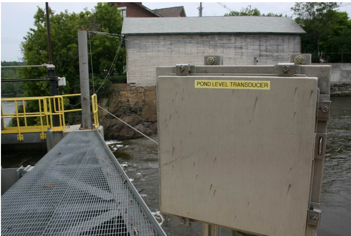
Photo 2. Pond level transducer.
