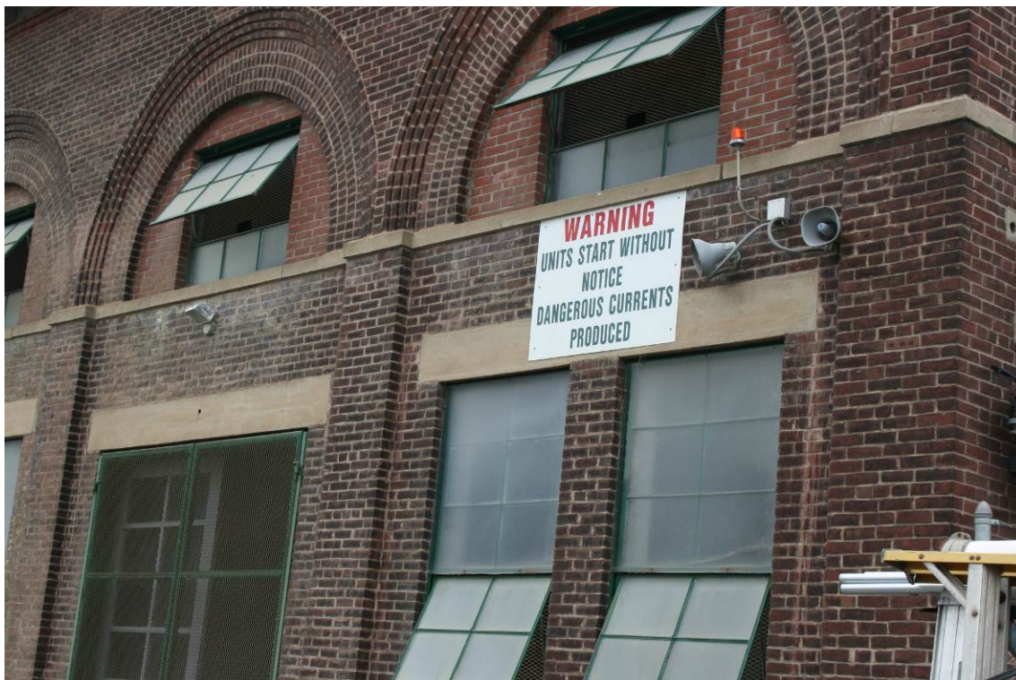
Photo 5. Safety signage on powerhouse 9 with strobe and sirens.
