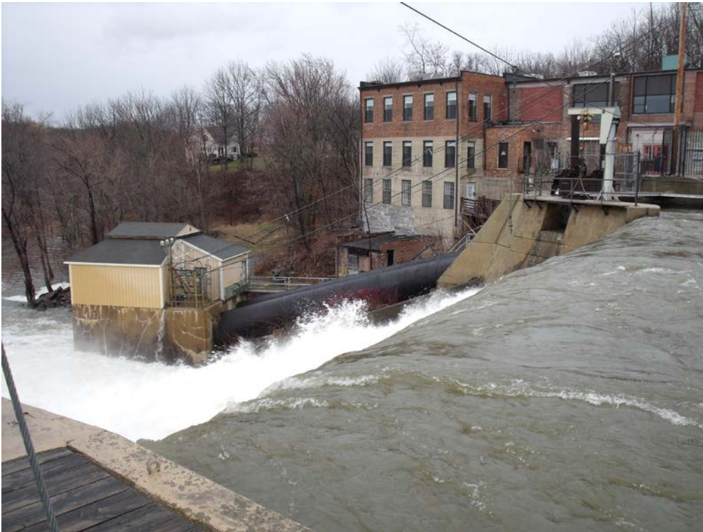
PHOTO 4 PLANT 9B INTAKE, PENSTOCKS, AND POWERHOUSE
