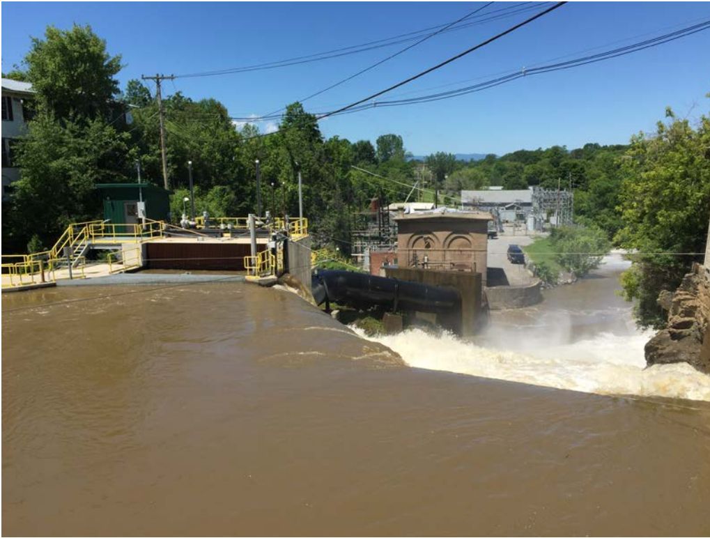
PHOTO 3 PLANT 9 INTAKE, PENSTOCKS, AND POWERHOUSE
