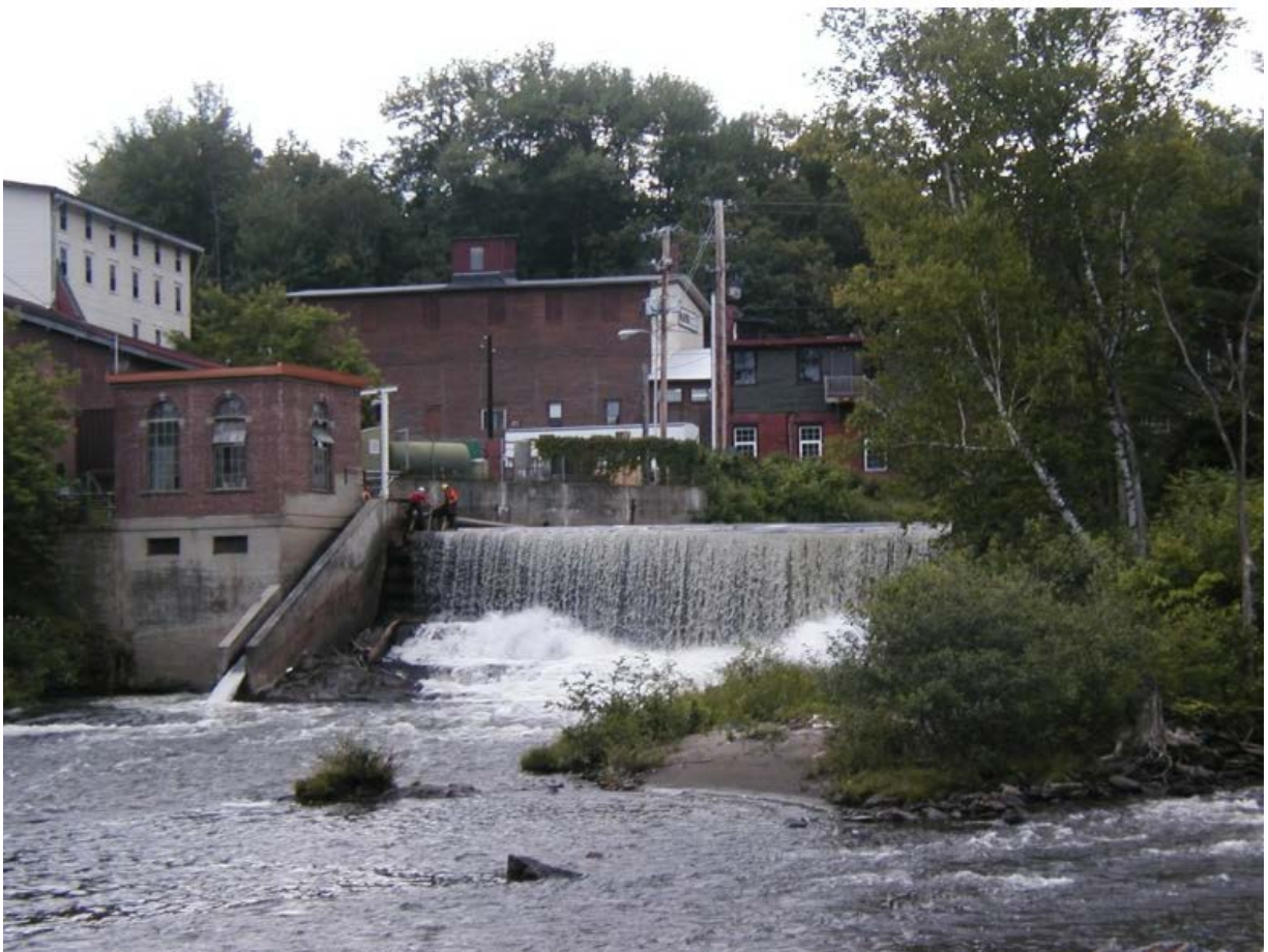
PHOTO 6 SOUTH DAM AND POWERHOUSE (NOTE SLUICeway BETWEEN SPILLWAY AND POWERHOUSE FOR DOWNSTREAM FISH PASSAGE AND MINIMUM FLOW RELEASES)
