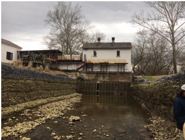
*Figure 11 Drained Forebay, Gabion embankment wall and trash racks*
