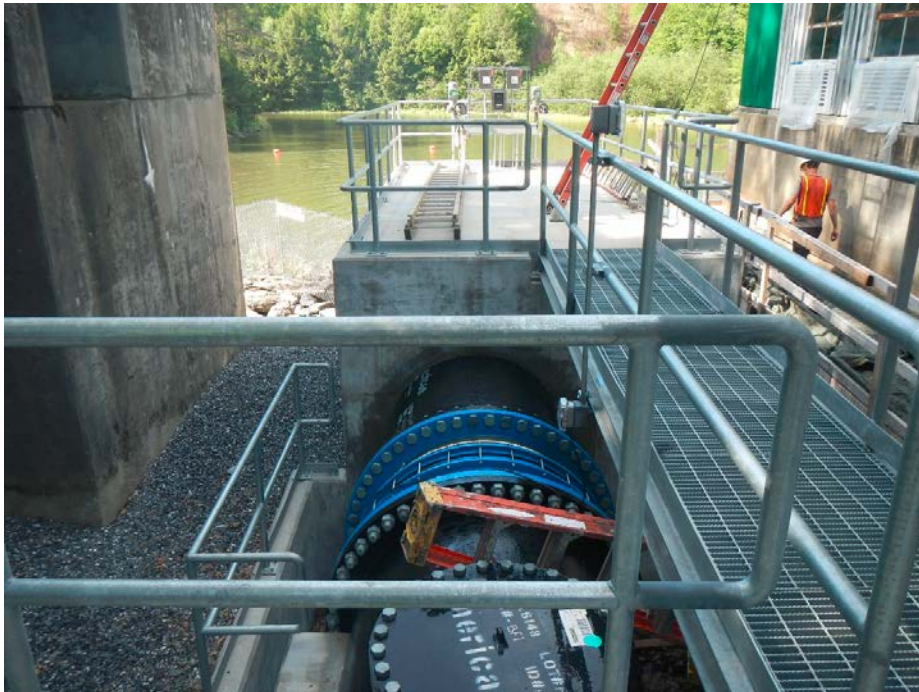
PHOTO 7 NEWLY INSTALLED FLOW DISCHARGE VALVES FOR STATION TRIPS OR UNIT SHUTDOWN.
