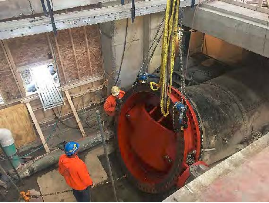
PHOTO 6 INSTALLING THE NEW 78" BUTTERFLY VALVE WITHIN THE WATERBURY POWERHOUSE FOR STAGE II OPERATIONS.
