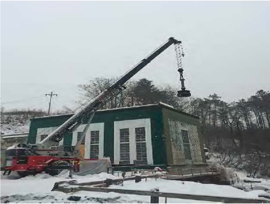
PHOTO 8 CRANE REMOVING EXISTING RUNNER FROM THE POWERHOUSE SO TO PREPARE FOR RUN-OF-RIVER OPERATIONS/STAGE II OPERATION.
