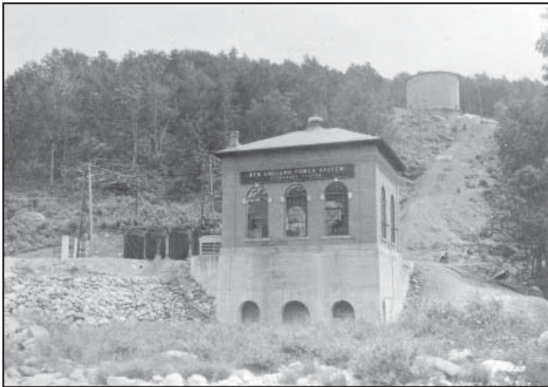
Searsburg Development, Searsburg, VT, built 1922. View looking south across Deerfield River showing surge tank (above) and powerhouse (below) (June 29, 1923 photo). Searsburg is a divided-fall facility, where the dam and powerhouse are separate. Water from the Searsburg dam is directed to the powerhouse through a 3.5-mile-long, banded wood stave penstock.
