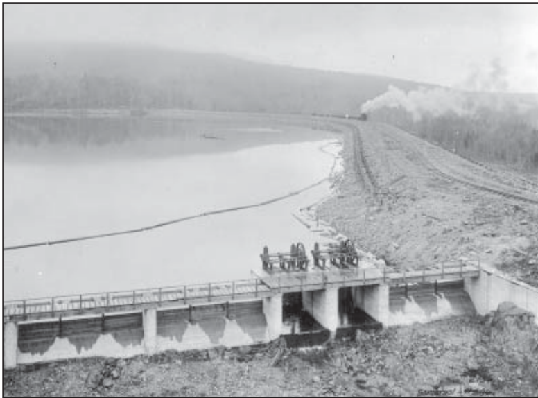
Somerset Development, Somerset, VT, built 1911–1913. View of 2,100-ft-long, 110-ft-high modified hydraulic earth fill dam looking south with spillway in foreground. Construction railway track and steam locomotive pulling dump cars are visible on dam crest (ca. 1913).
