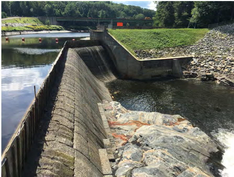
Photograph 8. No. 4 dam with flashboards on top and safety floats in distance. Vegetation at side of dam is maintained with herbicide. August 2018.
