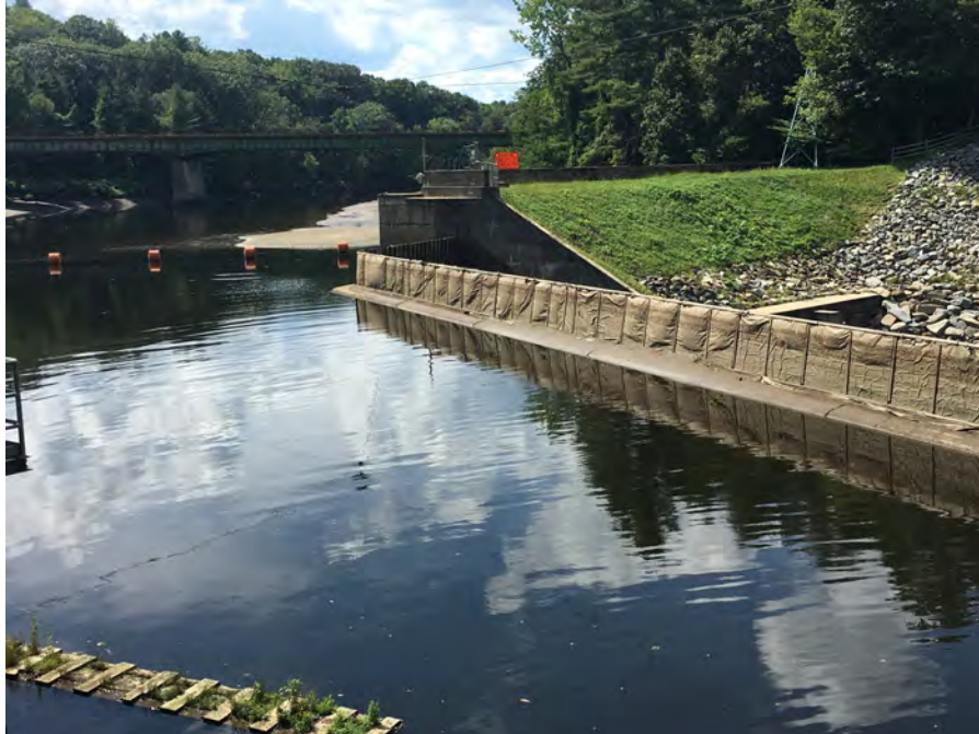
Photograph 7. View of debris boom in foreground, and plastic covered flashboards in distance. August 2018.
