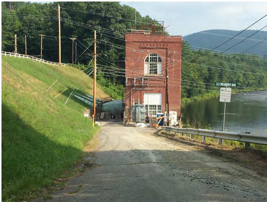
Photograph 12. The No.4 Station building requires ongoing maintenance. The vegetated slope is treated with herbicide to limit growth. August 2018.
