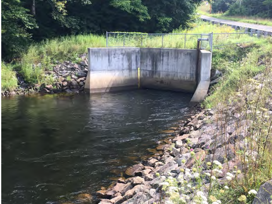
Photograph 5. Man-made canals convey water. The rip-rapped banks are maintained and treated with herbicide to restrict growth. August 2018.
