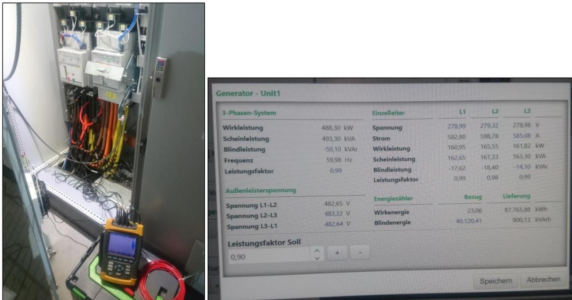
Figure 10: Control system Scada power measurement
