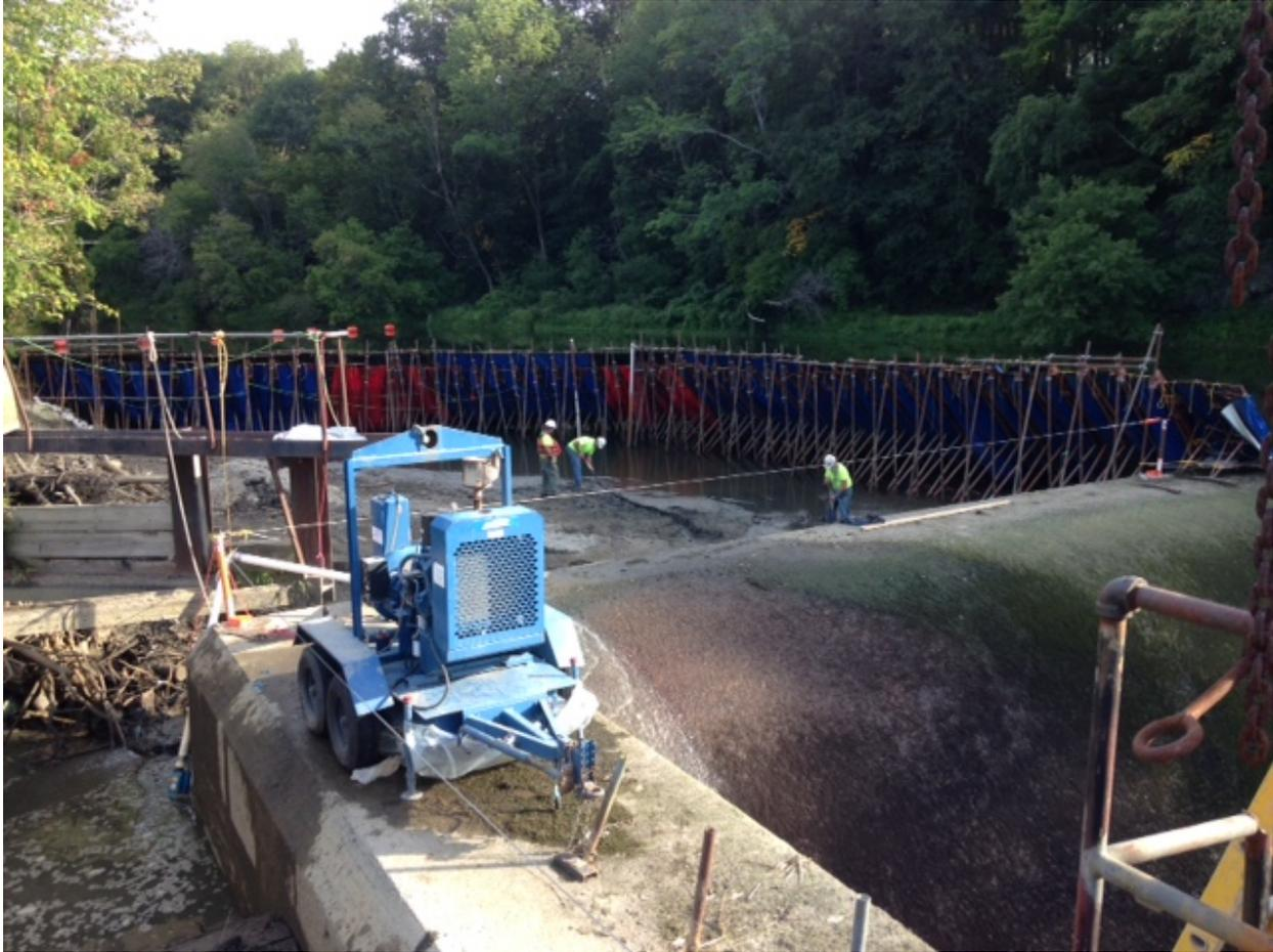
Figure 3. Pownal Dam dredging program to remove contaminated soil.
