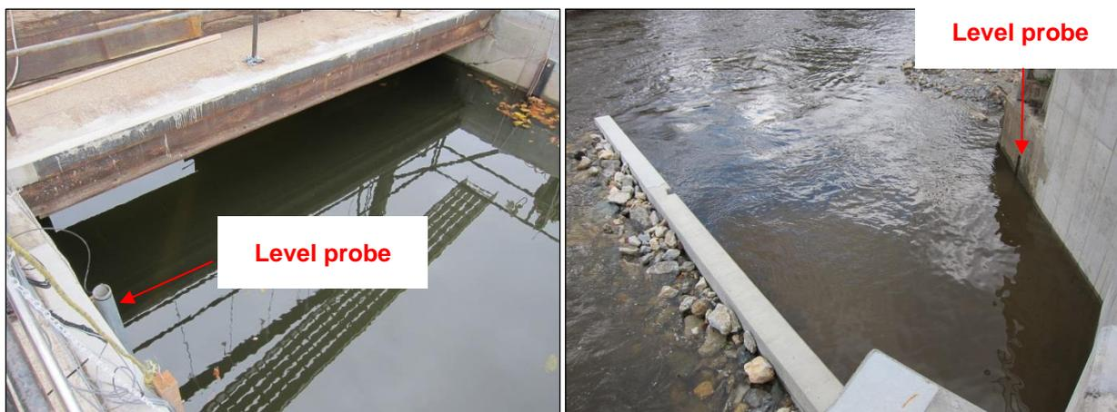
**Figure 9: Head and tail water measurement probe**
