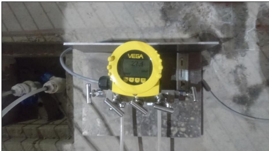
**Figure 12: Winter-Kennedy differential pressure measurement device**
