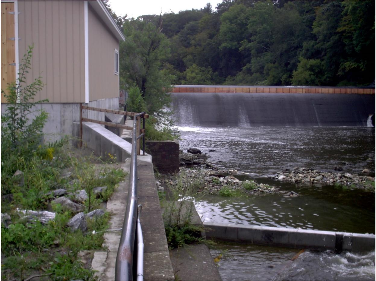
View of dam, powerhouse, tailrace, and bypass from right bank (note picture before new flashboard system was installed).
