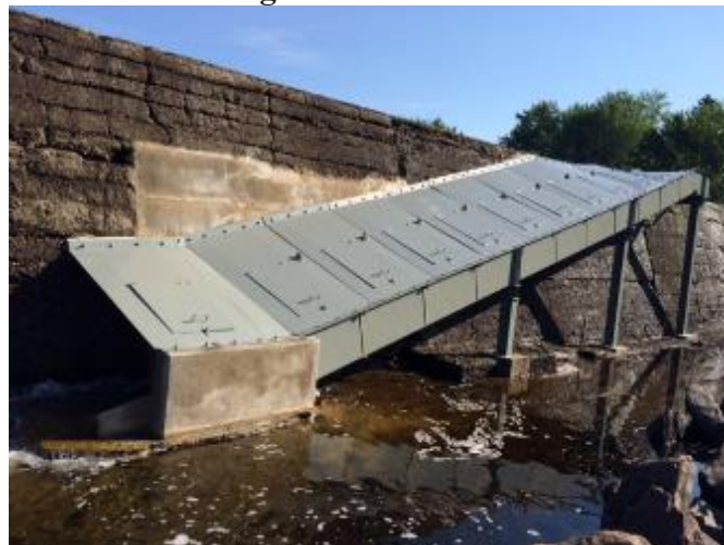
Figure 10 – Upstream Eel Ladder
