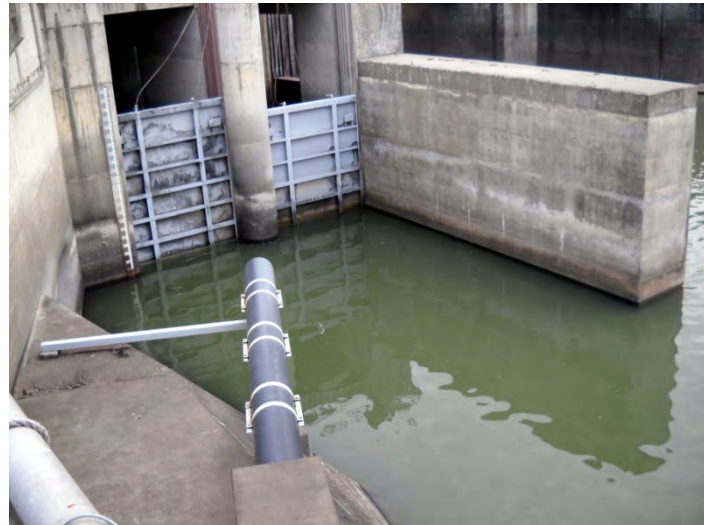
Figure 3. Fish bypass outfall at tailrace entrance to N1 ladder
