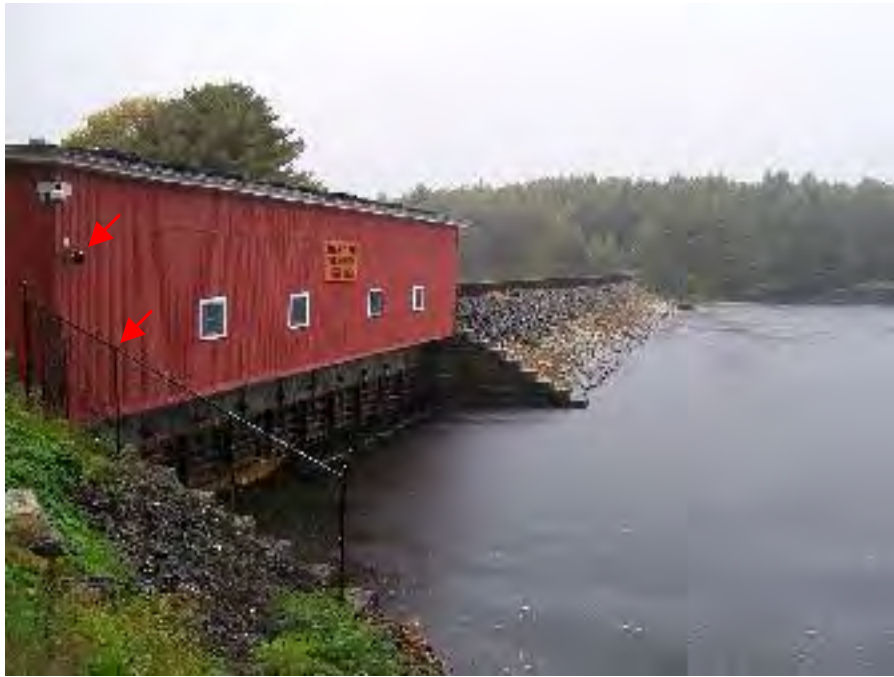
Photograph No. 3 - Headgate structure with warning sign. Note camera and fencing (arrow).
