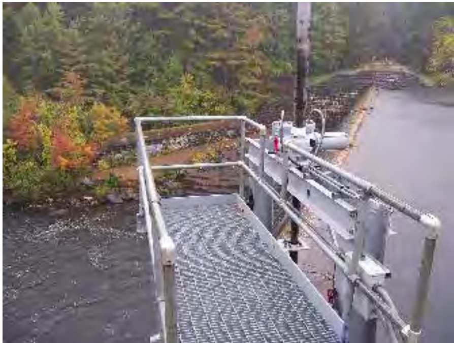
Photograph No. 2 - Gate release structure for minimum flow at dam.
