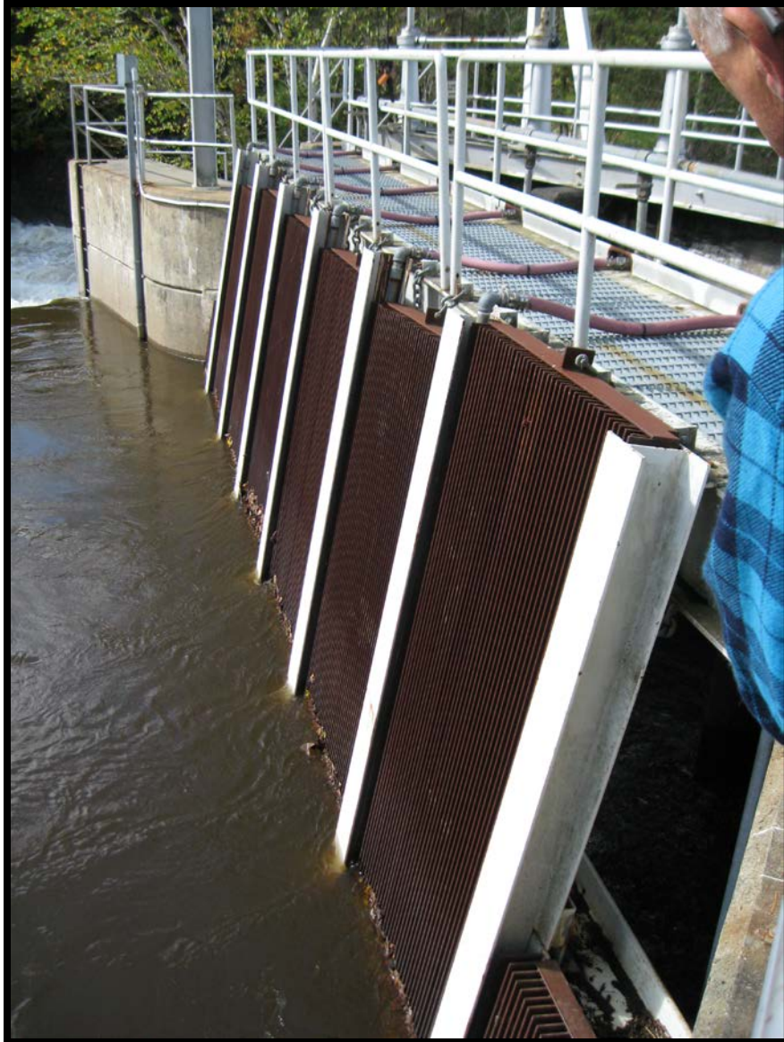
PHOTO 2 FISH DIVERSION RACKS AT HEAD OF POWER CANAL (NOW LOCATED IN FRONT OF THE INTAKE)
