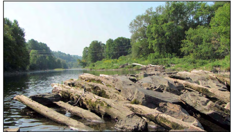
Location 7: Exposed timber crib dam ruins associated with Twin State Gas & Electric Co. No. 2 plant (1922-1944) within the Gage impoundment, looking south. August 31, 2010.
