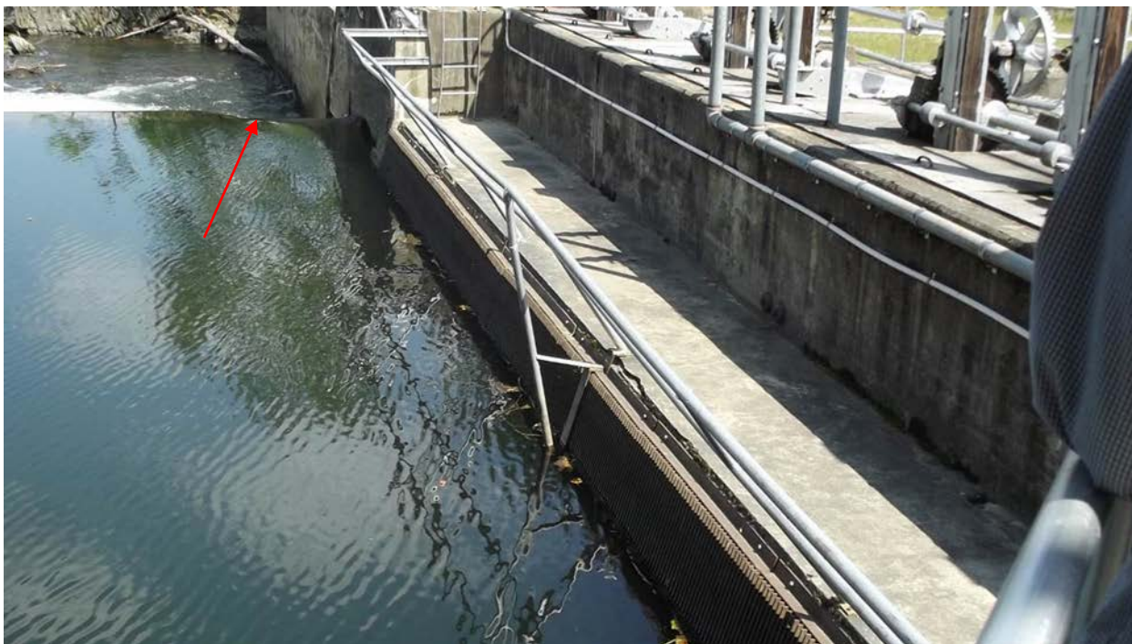
PHOTO 5 VIEW OF THE INTAKE WITH ONE-INCH, CLEAR-SPACED TRASHRACKS. NOTE SLUICEWAY FOR DOWNSTREAM FISH PASSAGE AND MINIMUM FLOW RELEASE (ARROW).
