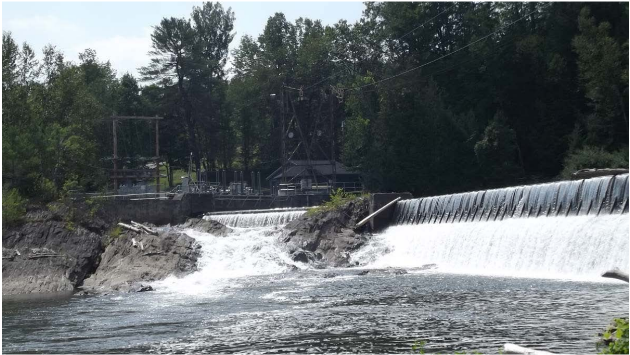
PHOTO 3 GAGE DAM VIEW OF THE SOUTH DAM (IN BACKGROUND) AND THE NORTH DAM (IN FOREGROUND) WITH HINGED FLASHBOARDS, SEPARATED BY A ROCK OUTCROPPING
