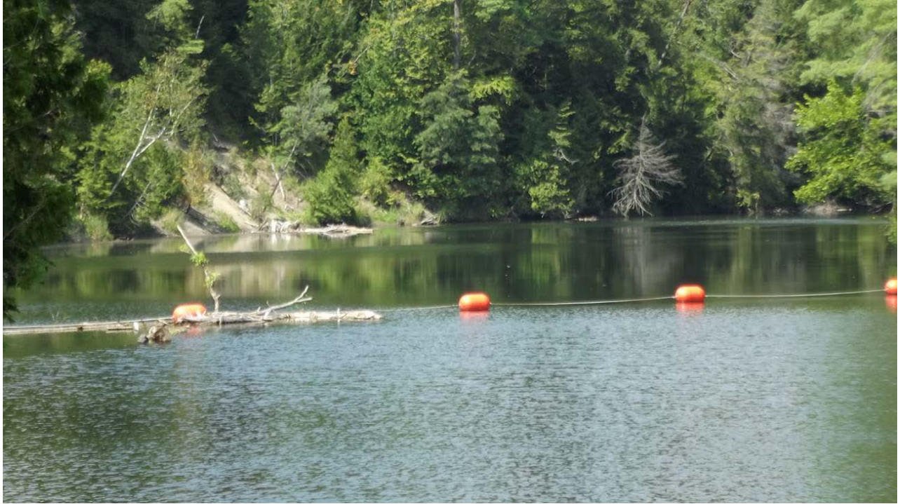
PHOTO 8 VIEW OF THE BOAT RESTRAINING BARRIER UPSTREAM OF THE DAMS
