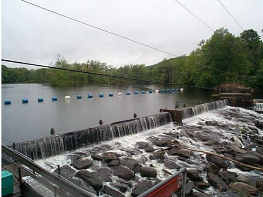
Figure 4 View of dam and impoundment from power station, showing boat safety barrier. (Source: 2001 FERC inspection report)
