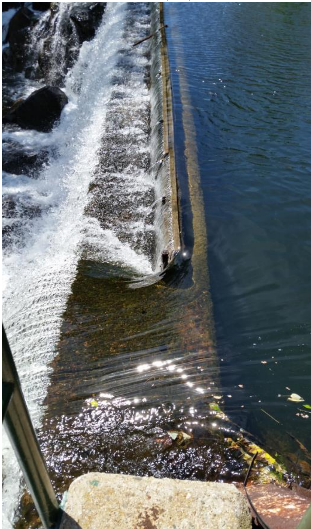
Flashboards removed for min flow section of spillway
