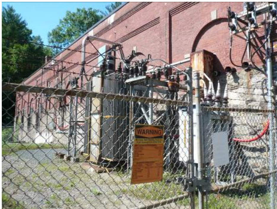
Photo 2: Project switchyard with warning signs and fencing (project was shut down at time of inspection). Note: most of the equipment shown is no longer in service as it has been replaced by equipment now located inside the powerhouse, and will likely be
