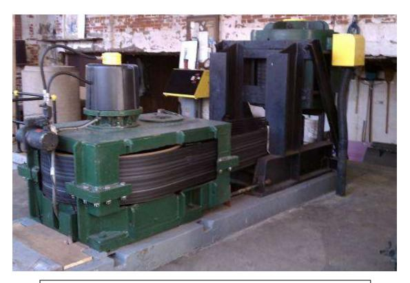
A belt driven Kaplan Turbine and Generator inside the Hydro Plant.
