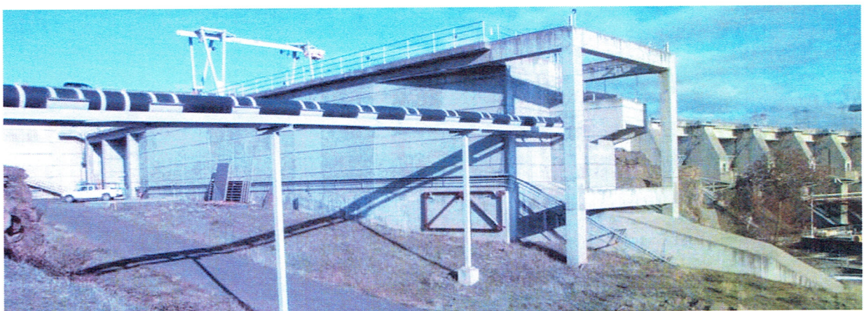
Photo 5. North side of dewatering structure and the bypass pipe that conveys fish to the tailrace.
