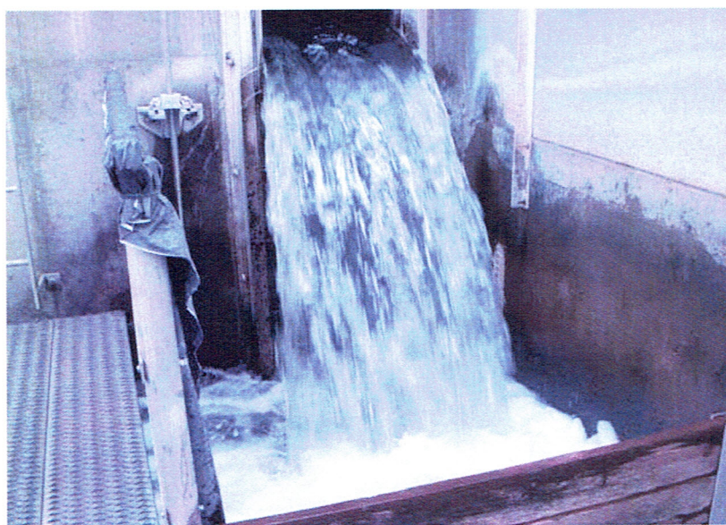
Photo 7. Weir discharge plunging into concrete basin.
