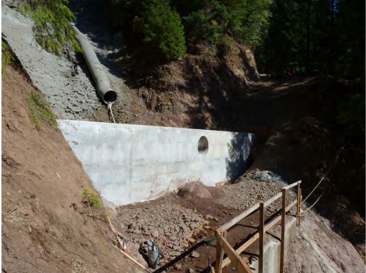
Figure 8. Concrete Toe Buttress
