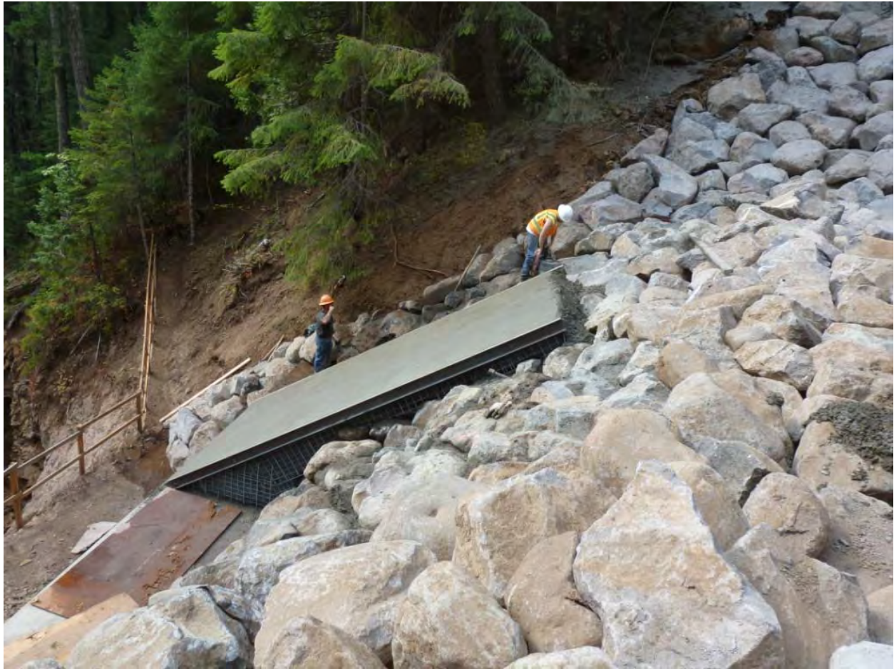
Figure 9. Grout filled rip rap and box culvert support
