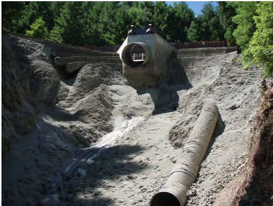
Photo 6- Wired and "shot-creted" channel; 7/27/11
