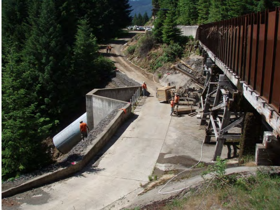
Photo 4- Drilling to install tie-backs to stabilize the “concrete transition structure”; 7/6/11
