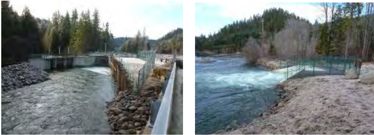
Figure 2.2-4 Lemolo No. 2 pipeline to Toketee Lake (inlet structure on left; outlet structure on right).
