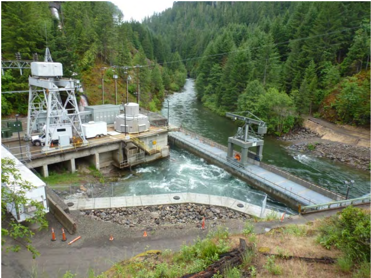
Figure 2.2-5 Slide Creek Powerhouse with tailrace barrier.
