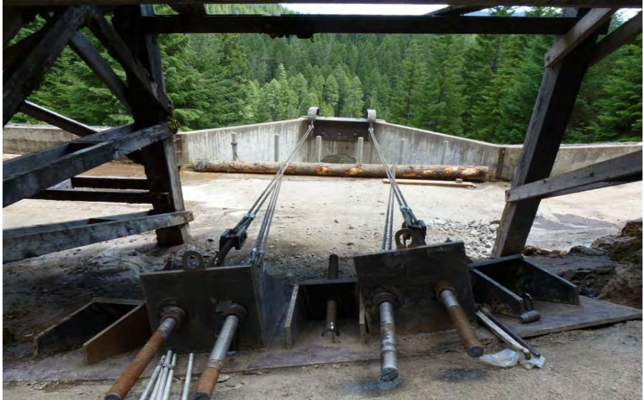
Figure 3. Transition Structure Tieback System
