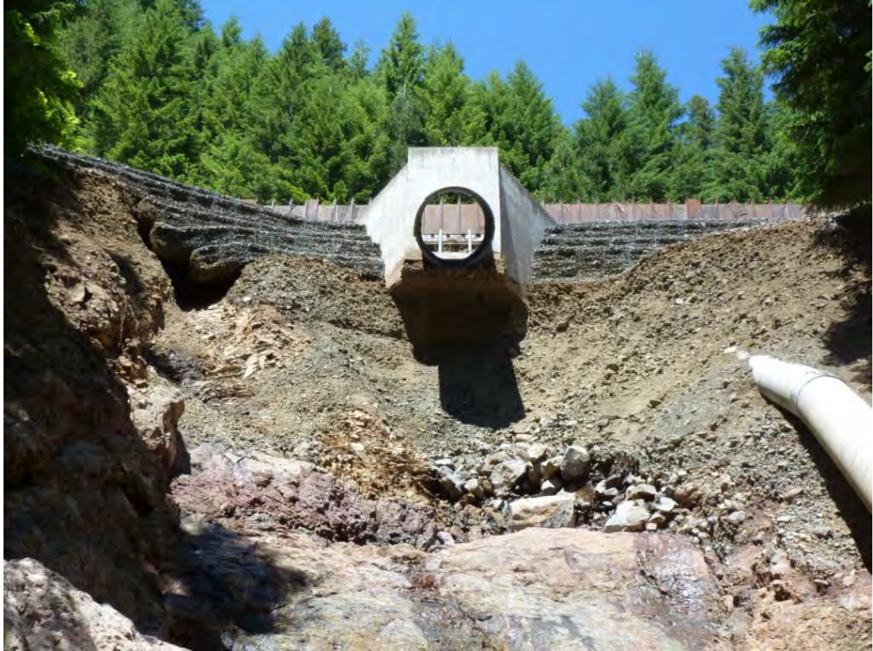
Figure 2. Erosion at Flume 12 Spillway
