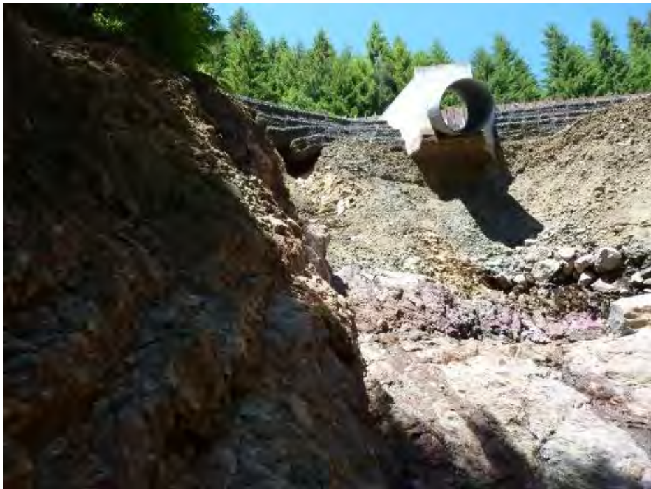
Photo 5- Concrete transition structure and origin of slide; looking up the slide route towards the Burma Road; 7/6/11
