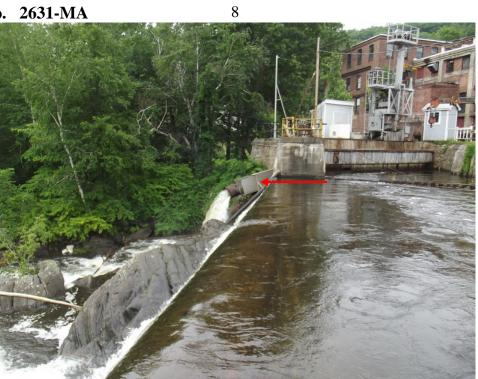
Photograph 5 - View looking at intake and downstream fish passage discharge pipe (arrow).
