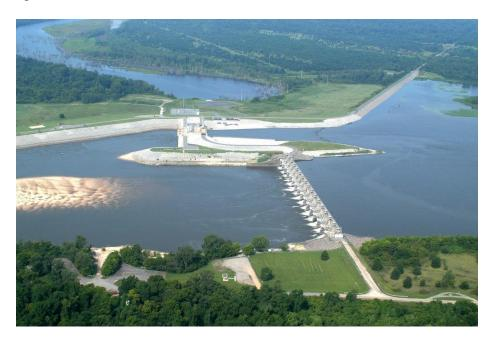
Aerial view looking west at Arkansas River Dam No. 2. The hydroelectric project, built into an existing non-overflow embankment, is to the west of the Corps spillway visible in foreground. The water body visible in the upper left of the photo is the old Arkansas River channel, cut off at the time Corps constructed the dam in the late 1960s, and fed by a water supply pipeline from the dam. See text for additional information.
