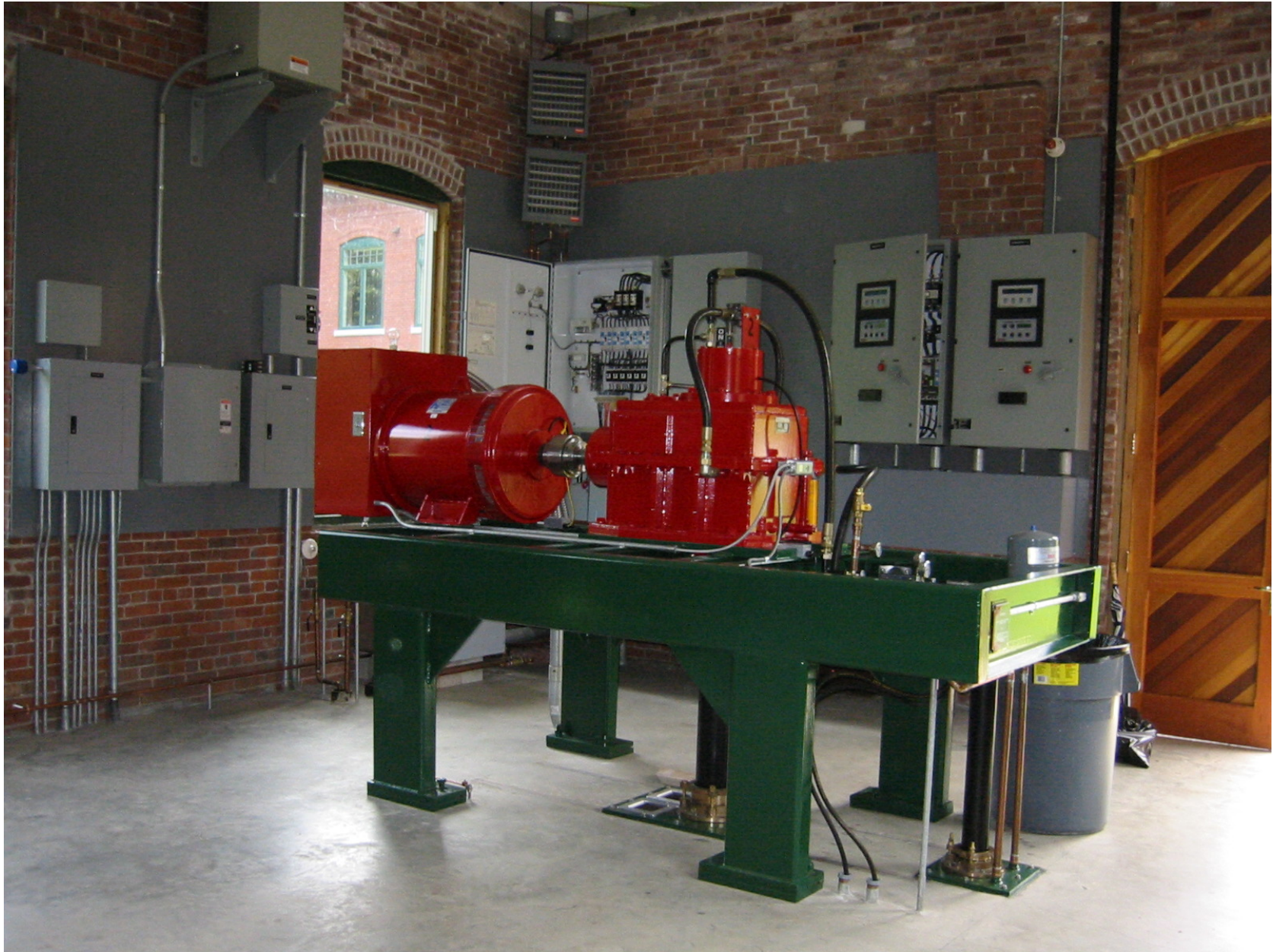
Ice House Partners, Attachment 12 - PHOTOS
