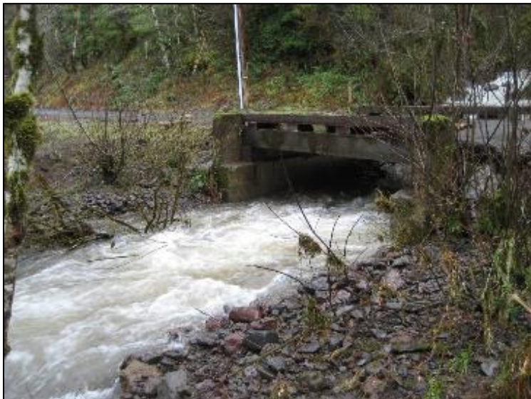
Figure 6: Falls Creek entering South Santiam River at FS Road 3024 at high water, river mile 56.
